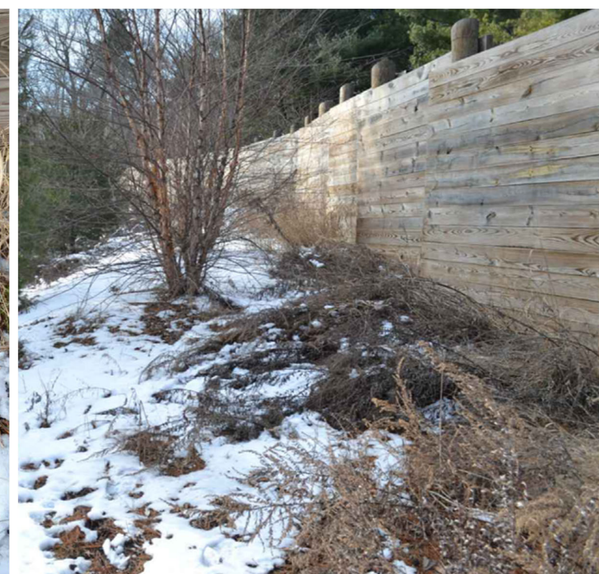
TYPICAL EXISTING WALL CHARACTER: 8' HIGH
