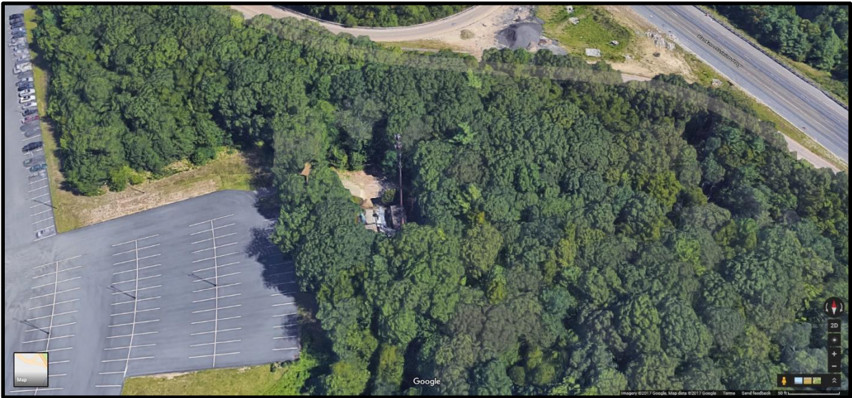
Figure 2: Existing Monopole (Center) Located at 100 Lowder Brook Drive, Westwood, MA (Picture courtesy Google Earth ©2017 and may not represent current conditions)
