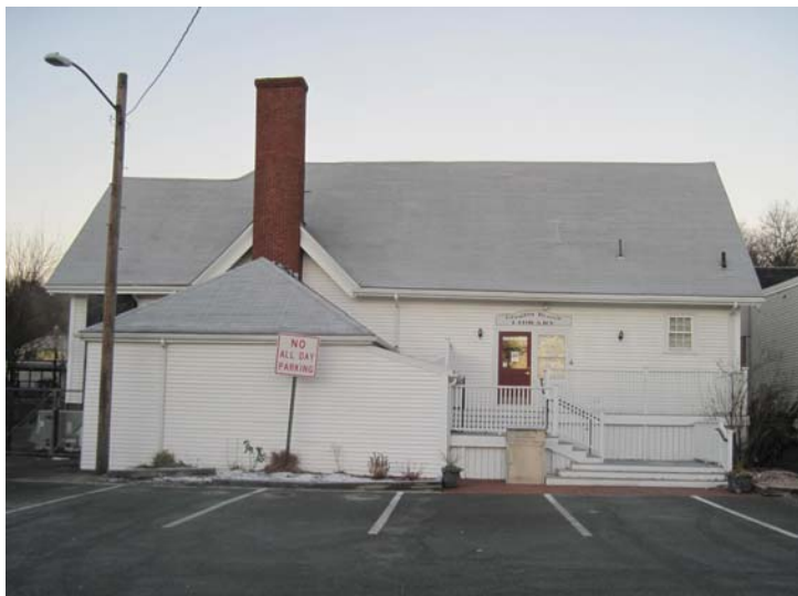
View of the rear (east) elevation with wood deck and stairs providing access to the rear entrance door.
