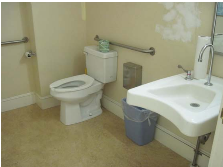
A fully-accessible bathroom is located just through the kitchen area. New vinyl sheet flooring was recently installed throughout the kitchen and bathroom in 2016.
