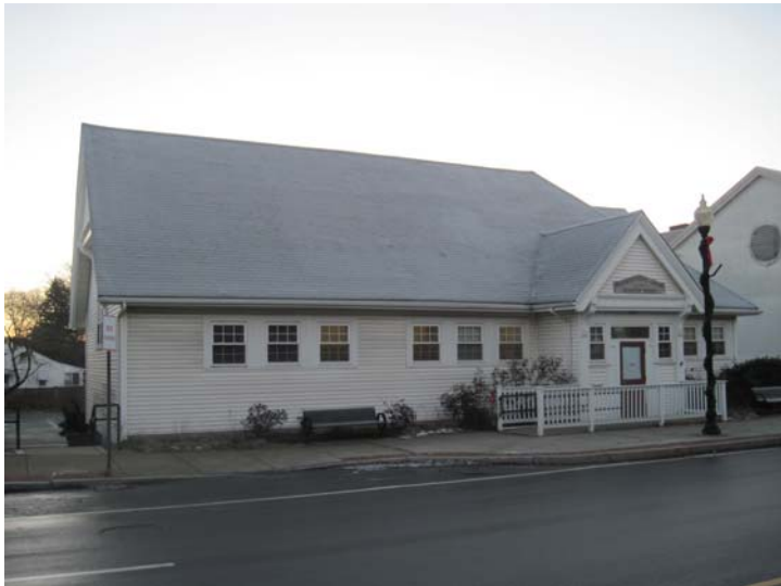
View of the building front (west) elevation with clapboard-profile vinyl siding and aging three-tab asphalt-shingle roof.
