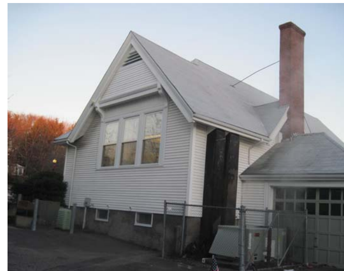
View of the south end-elevation
