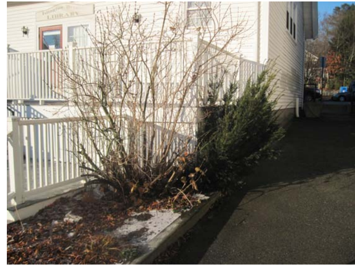
Overgrown shrubs adjacent to the rear-elevation deck are in need of trimming or removal.
