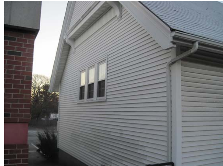
View of the building north end-elevation.
