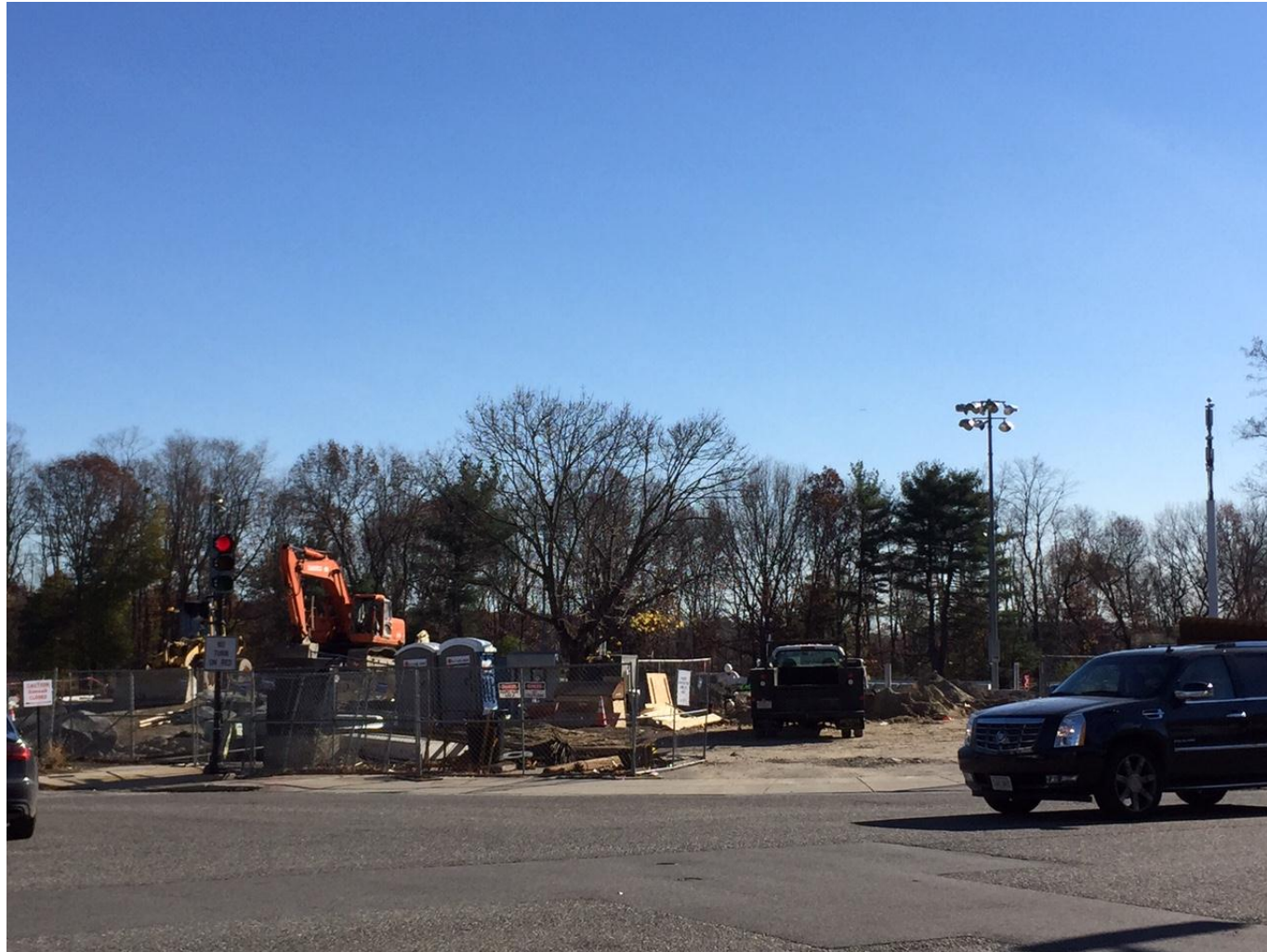
Under Construction - Islington Fire Station
