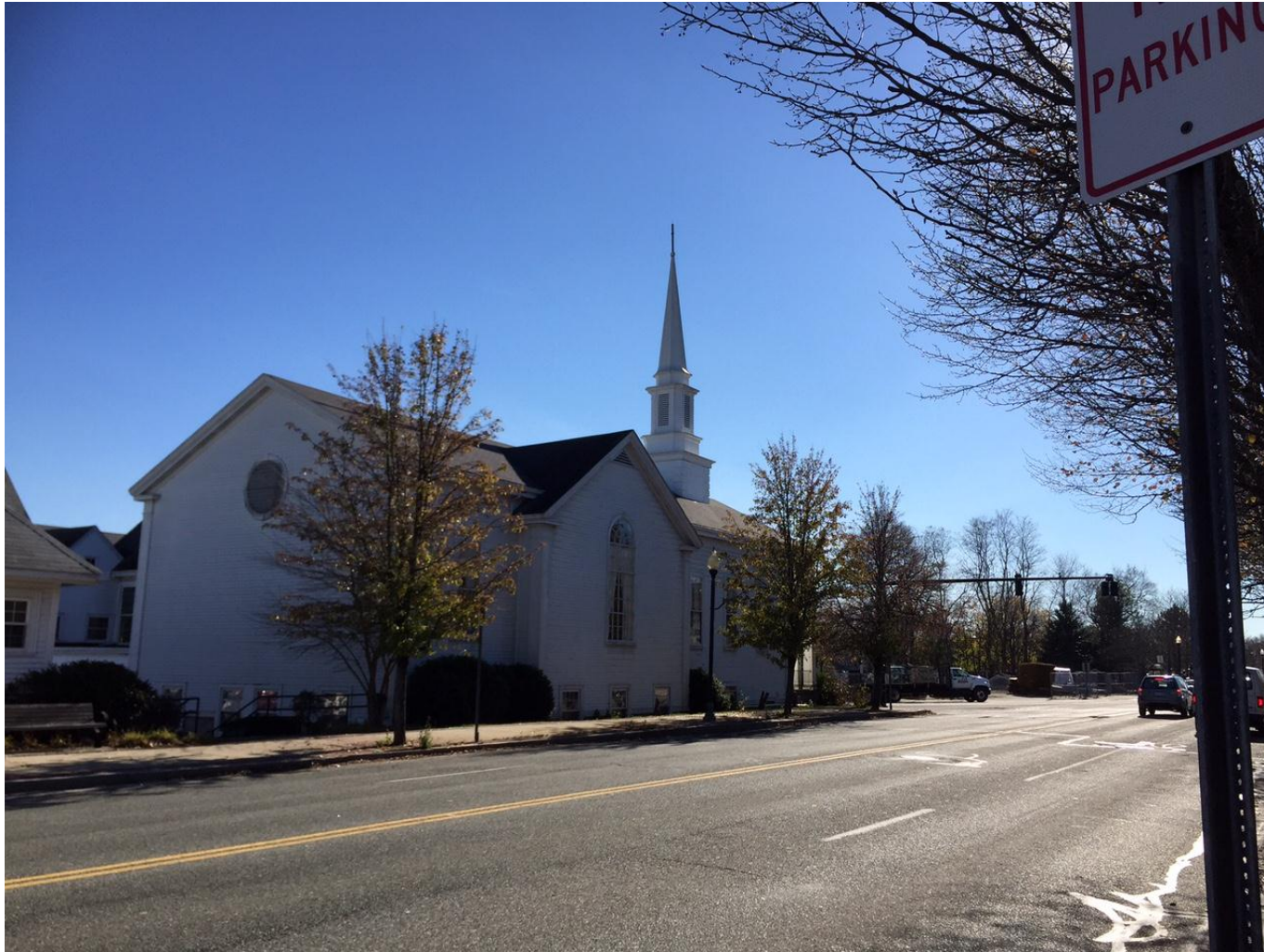
Islington Community Center – MMO Nursery School
