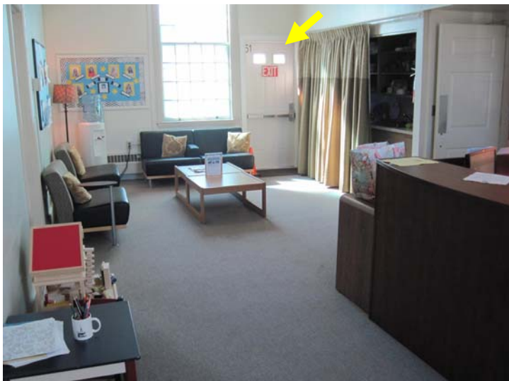
View of the second floor reception area finishes. Note newer accessible entry door accessed from the south elevation accessible entrance ramp
