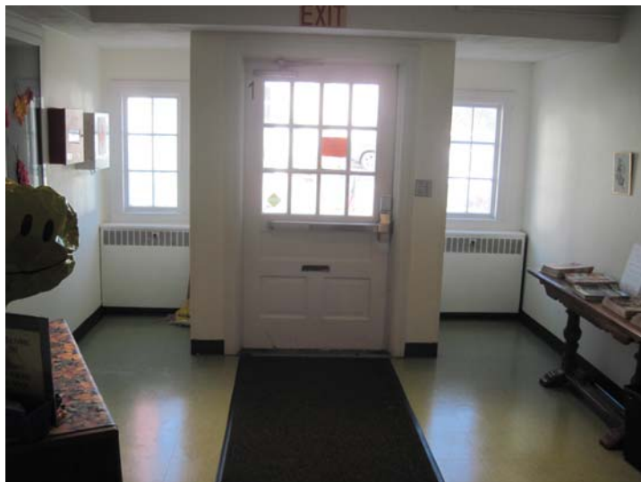
View of the front entrance hall finishes with painted walls and ceilings and VCT flooring.
