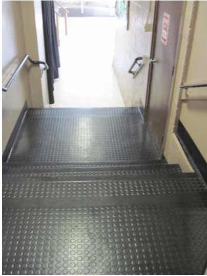
A set of stairs with raised-coin rubber treads and landings leads down to the large play hall.
