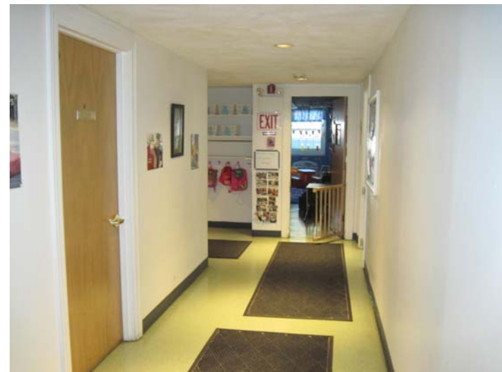
View of typical basement level hallway finishes.
