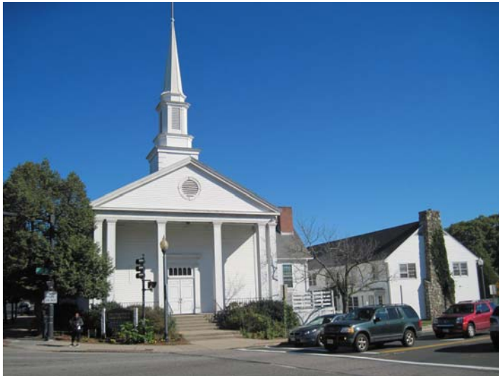
View of the building front (south) elevation. Original church structure at left with original painted-wood gutters and trim elements; and the 1960 addition at right with aluminum gutters and trim elements.
