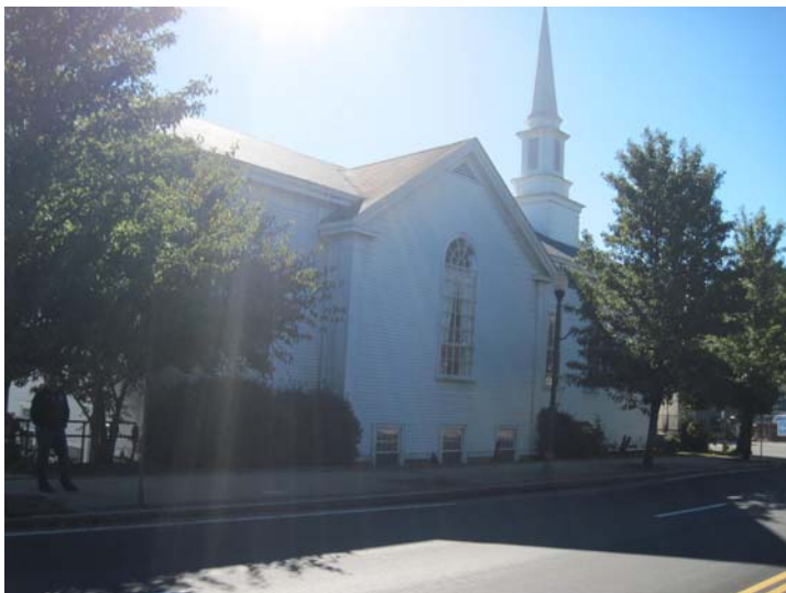
View of the building west elevation with original large wood-framed Palladian-style window.
