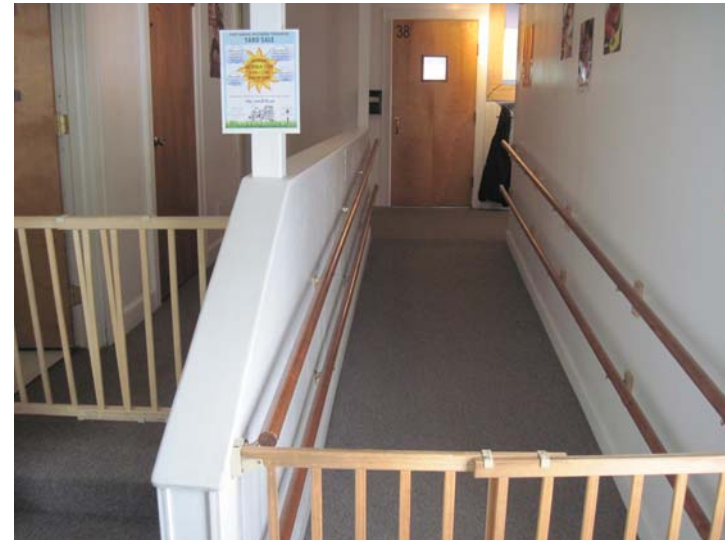
View of typical second floor hallway finishes with painted drywall walls and carpeted flooring.
