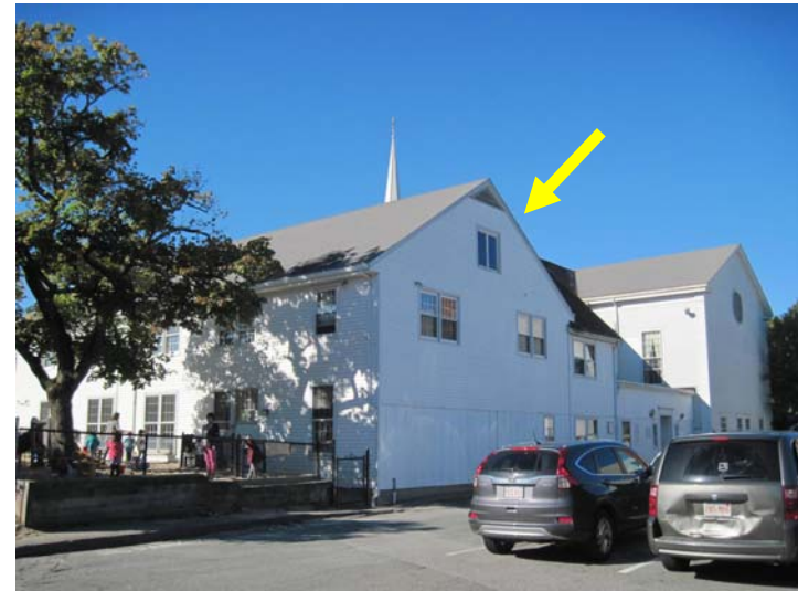
View of the building rear (north) elevation and east end-elevation. The section in the foreground (arrow) is an addition that was constructed in 1960.
