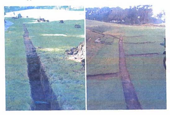
At the close of the day, the trench will be compacted, raked, and sod laid along the route of the irrigation lines. If sod was not salvaged from the path of the line, imported sod will be laid across the disturbed area. The goal is to restore the disturbed areas to a fully vegetated condition immediately.
