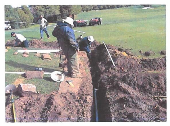
As the pipe is laid, and connections completed, the contractor will backfill the trench using the excavate along the side of the trench. Grassy areas will be raked and excess sediment removed from the work areas.
