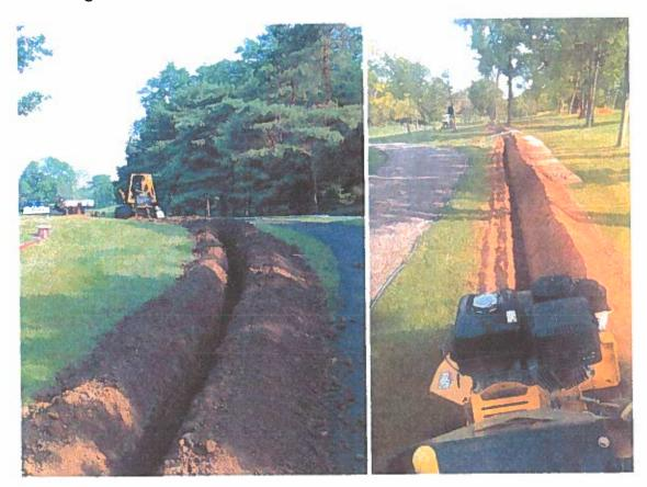
The digging of the new irrigation lines will be done with a mechanical trencher, a large-toothed blade attached to a small, tracked vehicle, such as a "Bobcat". (The common nomenclature is "Ditch Witch".) The installation requires a trench depth of approximately 18-36 inches. This can be done in a single pass of the trencher. The trencher lays the excavate along the edges of the trench, exposing the cut. After the trench is cut, the new HDPE lines will be laid, and the trench backfilled.
