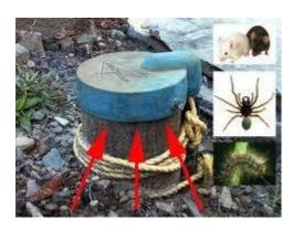
One of the best things a well owner can do regularly is to visually check the wellhead (the portion of the well above the surface) and the area around the wellhead. By doing so, you may detect potential issues before they become problems that jeopardize your water quality.
