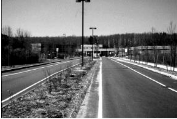
Reconstructed Rosemont Road in University Avenue Park.
