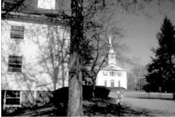
First Parish Church, Clapboard Tree Road.
