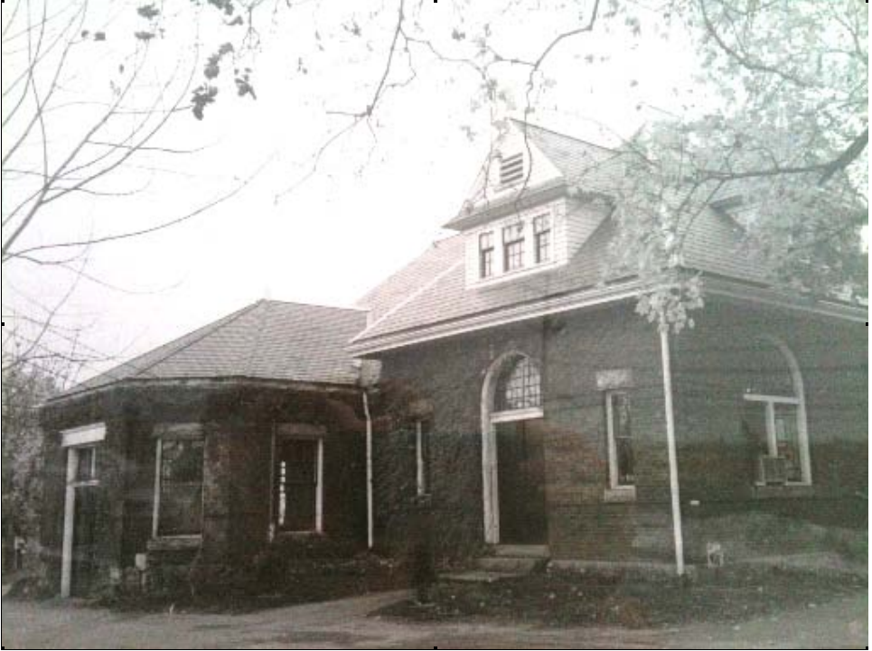
Bridge Street Treatment Plant and Pump Station
