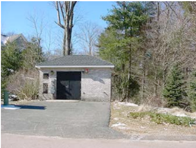
Pumping Station, Far Reach Road
