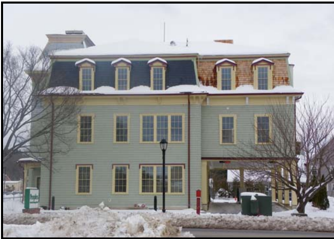
An addition to the rear elevation of the School accommodates a drive-thru for the bank, and additional space for the residential units above. Historic aspects of the original Colburn School have been added to the new addition, helping to unify the entire structure.
