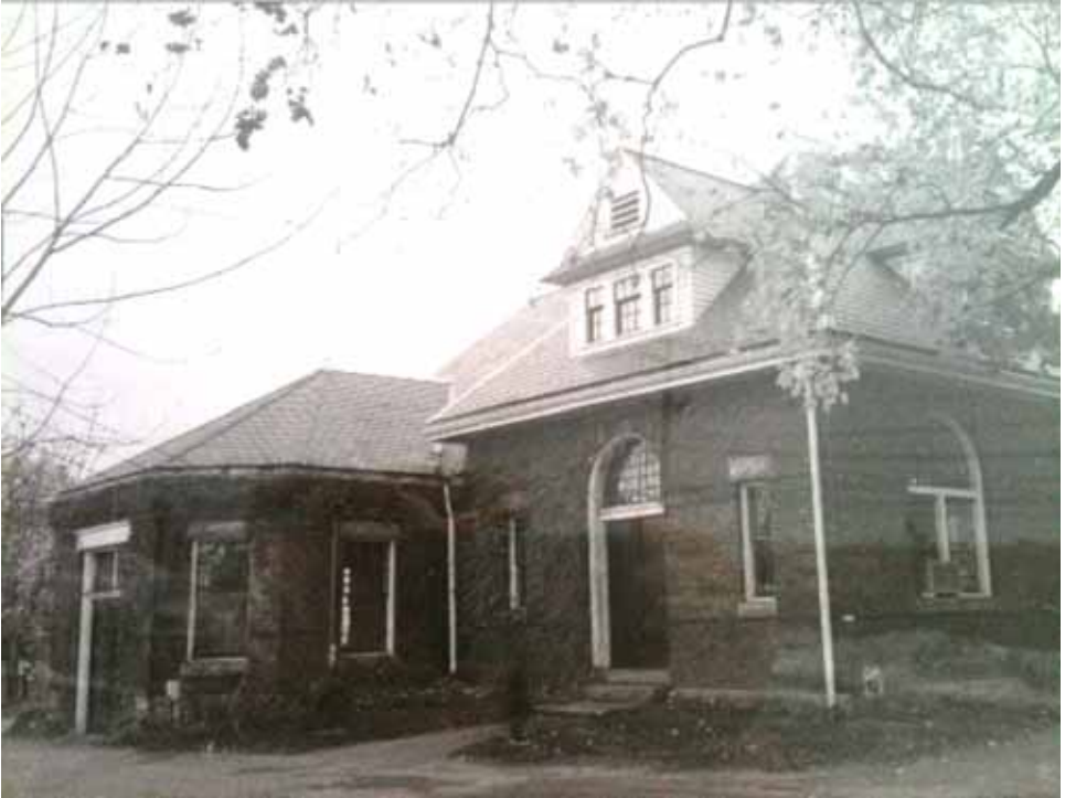
Bridge Street Treatment Plant and Pump Station
