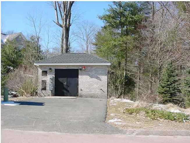
Pumping Station, Far Reach Road
