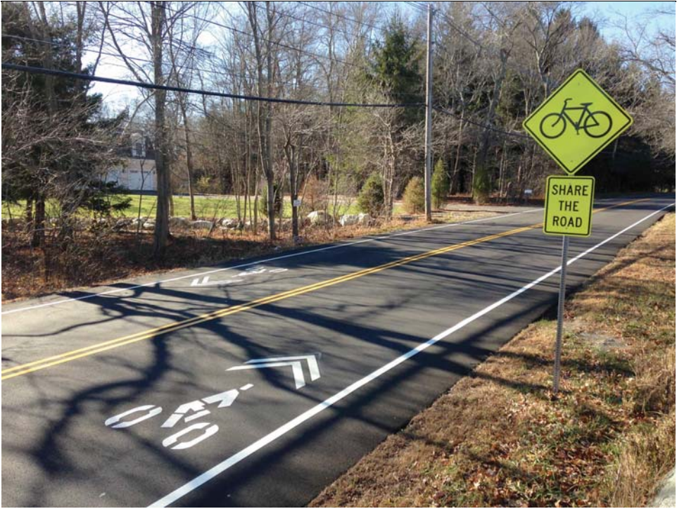
Westwood's first "share the road" arrows (also known as Sharrowes) incorporated into road improvements along Gay Street and Hartford Street
