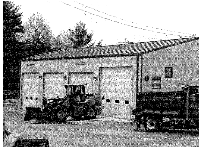
New Garage at Highway Yard
