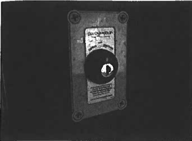
FIGURE 305.1(3) KEY SWITCH FOR POWERED POOL COVER OPERATION
