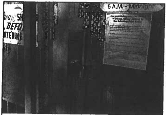
FIGURE 305.3.3(2) KEY CARD ENTRY ON GATE TO POOL AND SPA AREA MIGHT REQUIRE ALTERNATIVE METHOD APPROVAL
