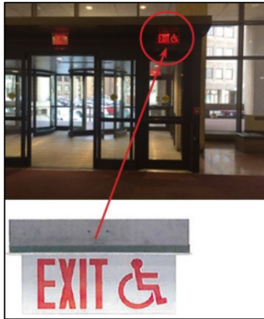
Illuminated exit sign with the International Symbol of Accessibility (ISA)
