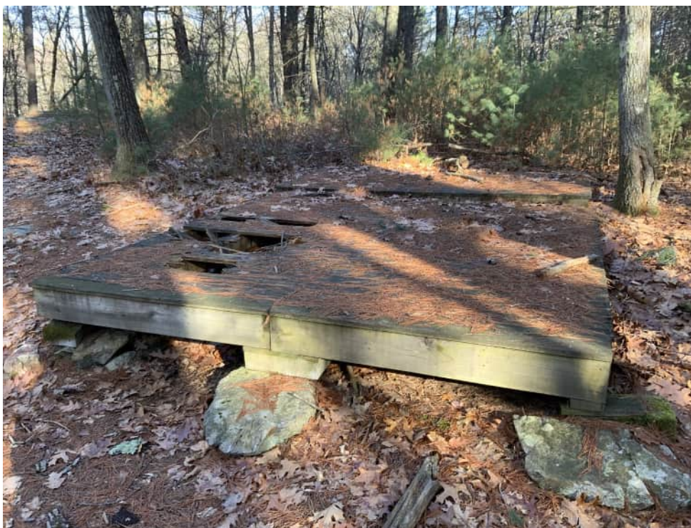
View of B1-107—facing south
