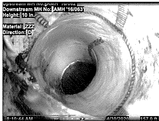
Photo 4: Looking up the sewer lateral from the sewer main
