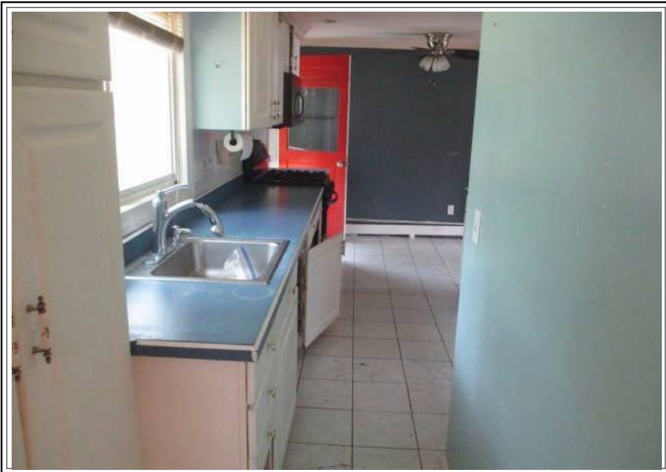
KITCHEN TO DINING AREA
