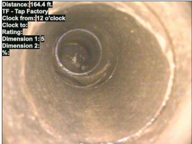
Photo: 15_033-15_034-20230801-104820.JPG At: 164.4 ft. 12/. TF - Tap Factory Joint: No
