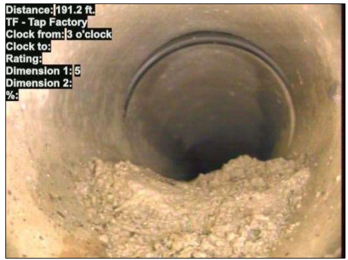
Photo: 15_077-15_078-20230801-072059.JPG At: 191.2 ft. 3/. TF - Tap Factory Joint: No
