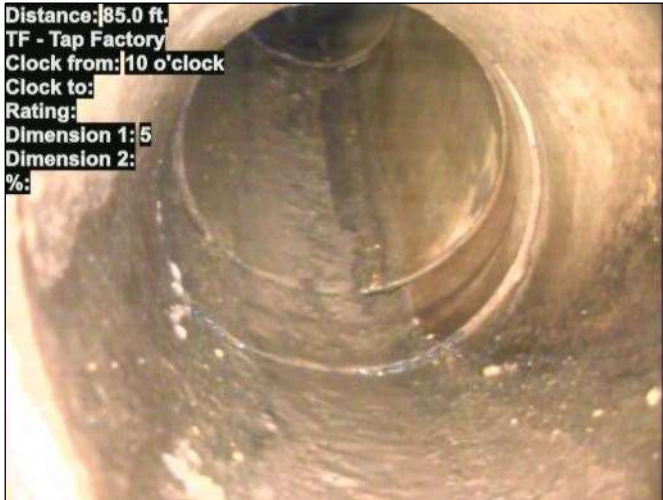
Photo: 15_057-15_046-20230725-081143.JPG At: 85 ft. 10/. TF - Tap Factory Joint: No
