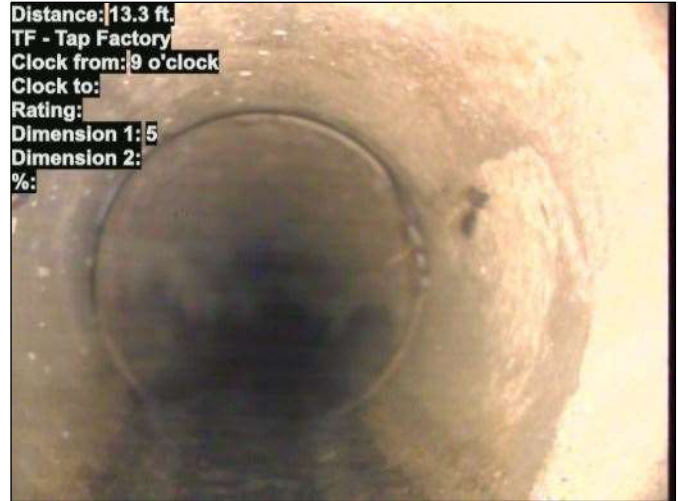
Photo: 15_077-15_078-20230801-071451.JPG At: 13.3 ft. 9/. TF - Tap Factory Joint: No
