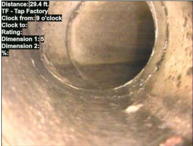
Photo: 15_028-15_029-20230724-163014.JPG At: 29.4 ft. 9/. TF - Tap Factory Joint: No
