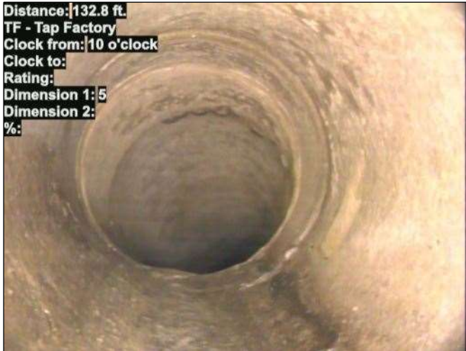
Photo: 15_050-15_051-20230726-070908.JPG At: 132.8 ft. 10/. TF - Tap Factory Joint: No
