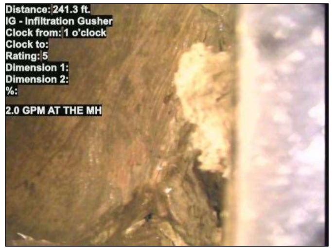
Photo: 15_047-15_048-20230725-094057.JPG At: 241.3 ft. 1/. IG - Infiltration Gusher Joint: No 2.0 GPM AT THE MH
