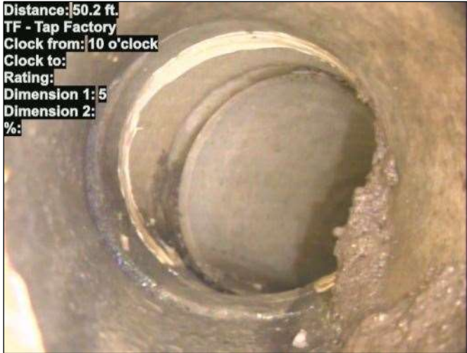
Photo: 15_013-15_014-20230725-124802.JPG At: 50.2 ft. 10/. TF - Tap Factory Joint: No
