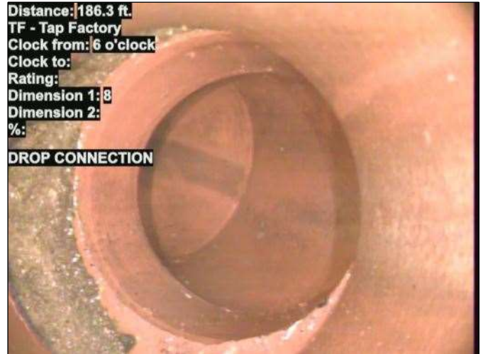
Photo: 15_049-15_050-20230726-064230.JPG At: 186.3 ft. 6/. TF - Tap Factory Joint: No DROP CONNECTION
