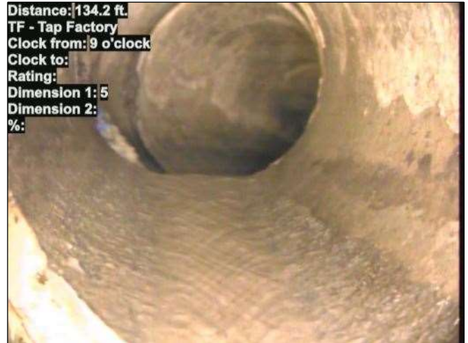
Photo: 15_027-15_026-20230725-183054.JPG At: 134.2 ft. 9/. TF - Tap Factory Joint: No
