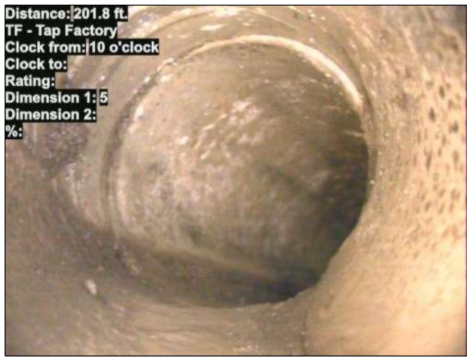
Distance: 201.8 ft. TF - Tap Factory Clock from: 10 o'clock Clock to: Rating: Dimension 1: 5 Dimension 2: %: Photo: 15_028-15_029-20230724-163643.JPG At: 201.8 ft. 10/. TF - Tap Factory Joint: No
