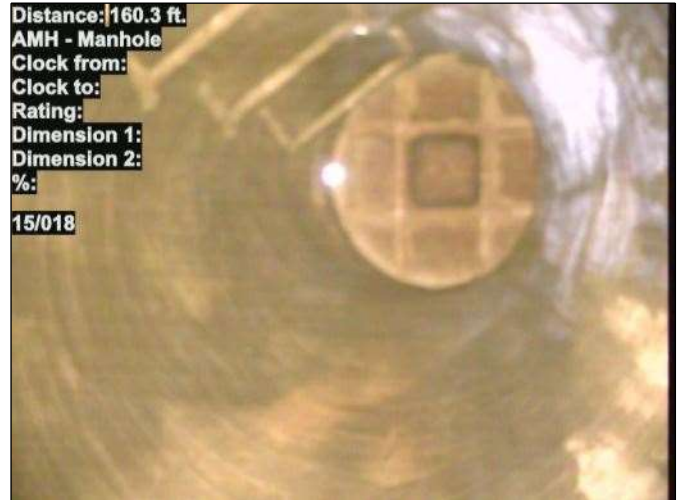
Photo: 15_017-15_018-20230724-150929.JPG At: 160.3 ft. AMH - Manhole Joint: No 15/018
