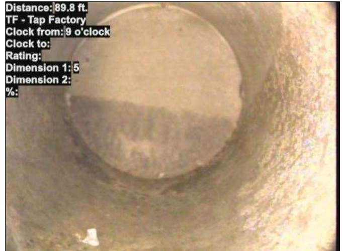
Photo: 15_019-15_018-20230721-114524.JPG At: 89.8 ft. 9/. TF - Tap Factory Joint: No
