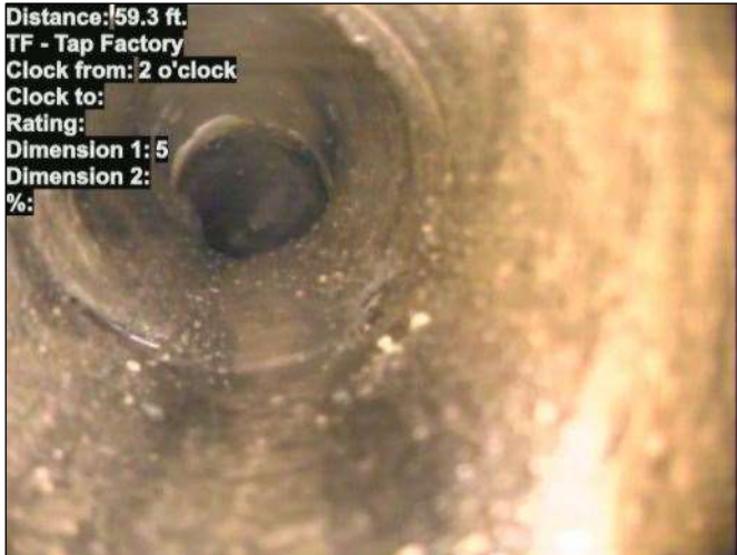
Photo: 15_025-15_024-20230801-100111.JPG At: 59.3 ft. 2/. TF - Tap Factory Joint: No
