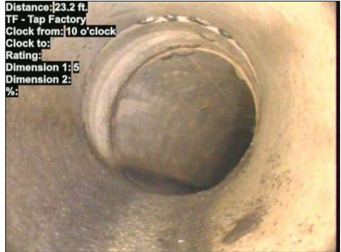
Photo: 15_044-15_045-20230725-085537.JPG At: 23.2 ft. 10/. TF - Tap Factory Joint: No
