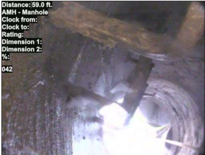
Photo: 15_041-15_042-20230801-124233.JPG At: 59 ft. AMH - Manhole Joint: No 042
