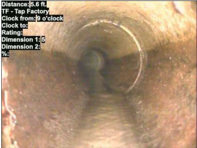
Photo: 15_073-15_072-20230726-073132.JPG At: 5.6 ft. 9/. TF - Tap Factory Joint: No
