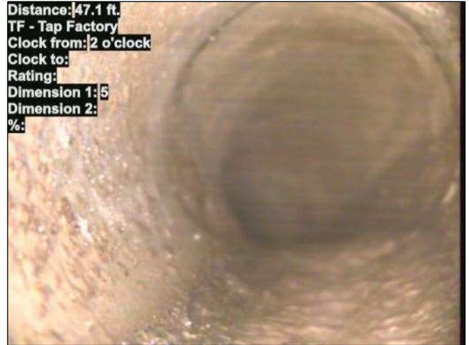
Photo: 15_020-15_021-20230724-152430.JPG At: 47.1 ft. 2/. TF - Tap Factory Joint: No
