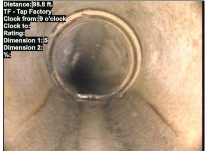
Photo: 15_073-15_072-20230726-073444.JPG At: 98.8 ft. 9/. TF - Tap Factory Joint: No
