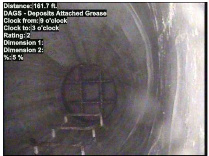
Photo: 15_043-15_058-20230804-072530.JPG At: 161.7 ft. 9/3 DAGS - Deposits Attached Grease Joint: No 5 %
