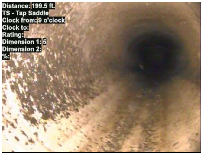
Photo: 15_037-15_038-20230724-122631.JPG At: 199.5 ft. 9/. TS - Tap Saddle Joint: No
