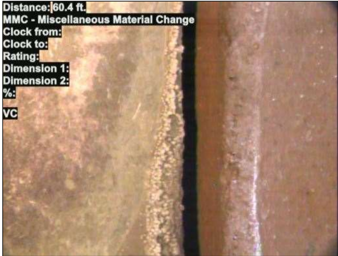
Photo: 15_032-15_033-20230725-071659.JPG At: 60.4 ft. MMC - Miscellaneous Material Change Joint: No VC
