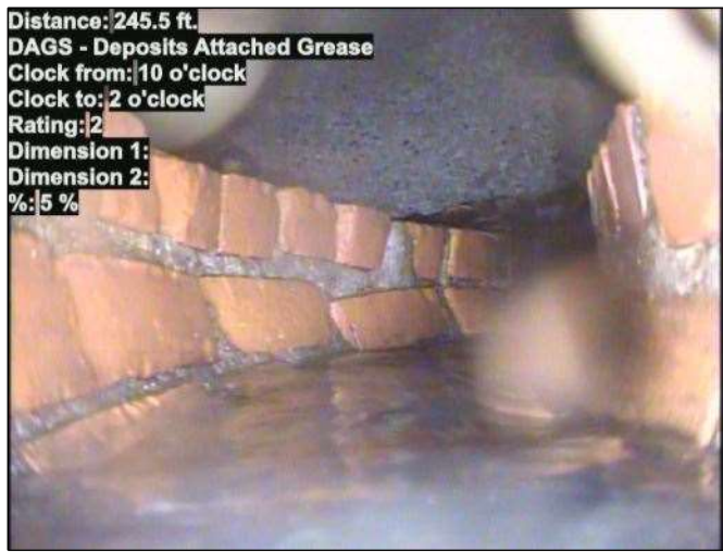
Photo: 15_059-15_060-20230804-090132.JPG At: 245.5 ft. DAGS - Deposits Attached Grease 10/2 Joint: No 5 %
