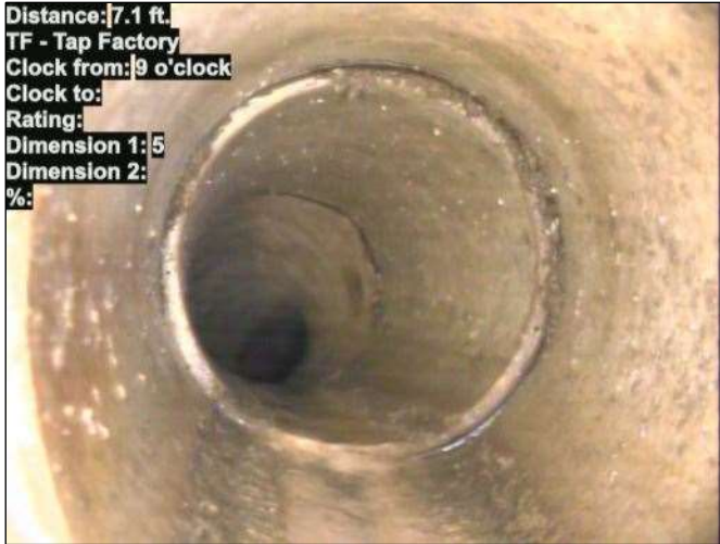
Photo: 15_027-15_026-20230725-182351.JPG At: 7.1 ft. 9/. TF - Tap Factory Joint: No
