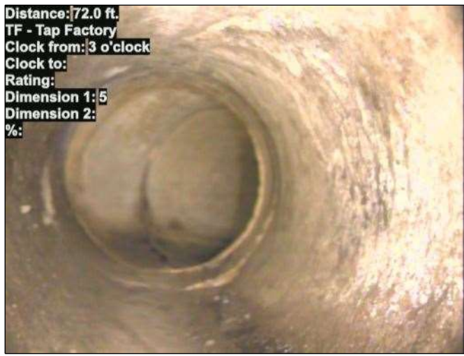
Photo: 15_048-15_033-20230725-103851.JPG At: 72 ft. 3/. TF - Tap Factory Joint: No
