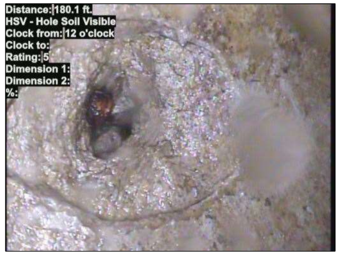
Photo: 15_059-15_060-20230804-085823.JPG At: 180.1 ft. 12/. HSV - Hole Soil Visible Joint: No
