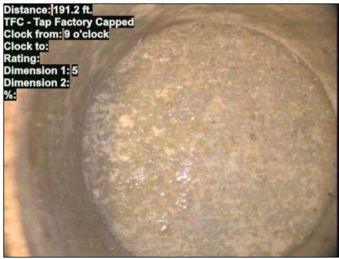
Photo: 15_031-15_032-20230724-170524.JPG At: 191.2 ft. 9/. TFC - Tap Factory Capped Joint: No
