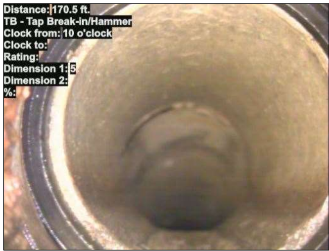
Distance: 170.5 ft. TB - Tap Break-in/Hammer Clock from: 10 o'clock Clock to: Rating: Dimension 1: 5 Dimension 2: %: Photo: 15_016-15_017-20230724-140931.JPG At: 170.5 ft. 10/. TB - Tap Break-in/Hammer Joint: No
