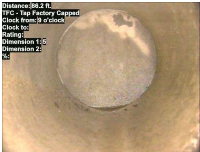
Photo: 15_048-15_033-20230725-103955.JPG At: 86.2 ft. 9/. TFC - Tap Factory Capped Joint: No
