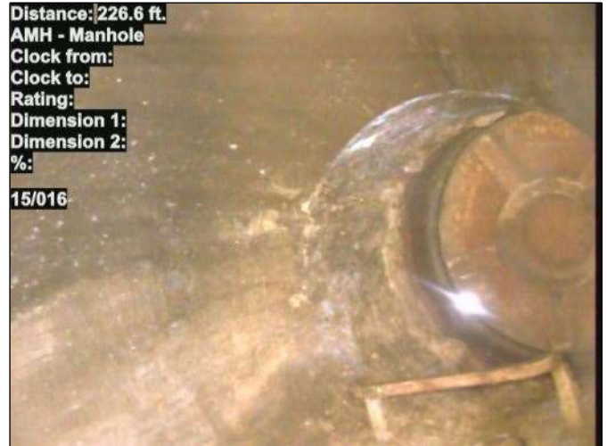
Photo: 15_015-15_016-20230724-135816.JPG At: 226.6 ft. AMH - Manhole Joint: No 15/016
