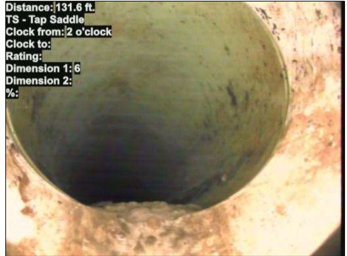
Photo: 15_001-15_002-20230725-122140.JPG At: 131.6 ft. 2/. TS - Tap Saddle Joint: No
