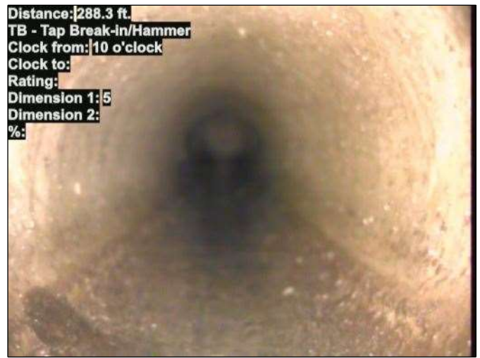
Photo: 15_037-15_038-20230724-122854.JPG At: 288.3 ft. 10/. TB - Tap Break-in/Hammer Joint: No
