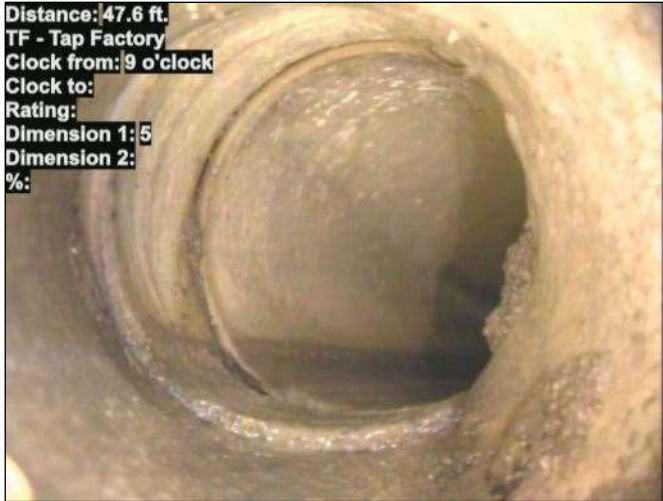
Photo: 15_037-15_038-20230724-121808.JPG At: 47.6 ft. 9/. TF - Tap Factory Joint: No
