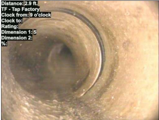
Photo: 15_025-15_024-20230801-095807.JPG At: 2.9 ft. 9/. TF - Tap Factory Joint: No
