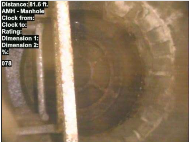
Photo: 15_079-15_078-20230801-081727.JPG At: 81.6 ft. AMH - Manhole Joint: No 078
