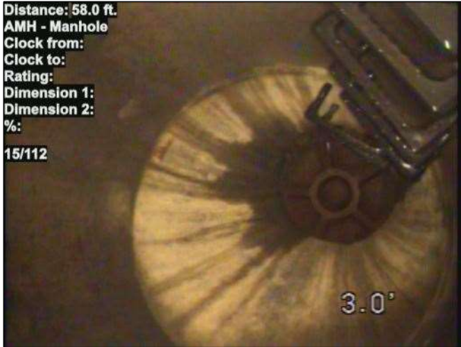
Photo: 15_112-15_005-20230807-104202.JPG At: 58 ft. AMH - Manhole Joint: No 15/112
