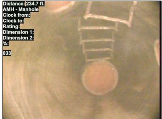
Photo: 15_024-15_033-20230801-101754.JPG At: 234.7 ft. AMH - Manhole Joint: No 033
