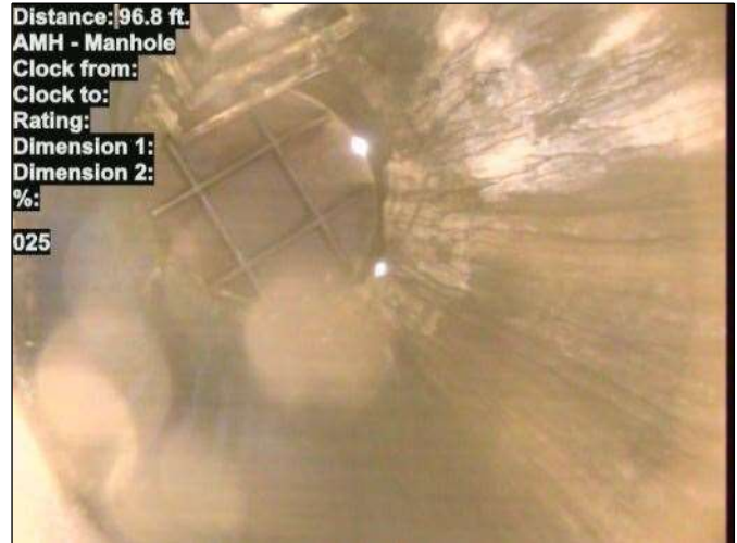
Photo: 15_018-15_025-20230801-095321.JPG At: 96.8 ft. AMH - Manhole Joint: No 025
