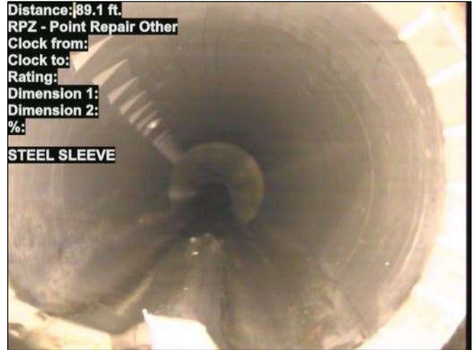
Photo: 15_071-15_072-20230726-082330.JPG At: 89.1 ft. RPZD - Point Repair Other Defective Joint: No STEEL SLEEVE
