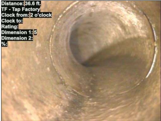
Photo: 15_023-15_024-20230724-155519.JPG At: 36.6 ft. 2/. TF - Tap Factory Joint: No
