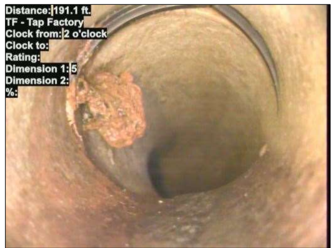
Photo: 15_022-15_023-20230724-155104.JPG At: 191.1 ft. 2/. TF - Tap Factory Joint: No
