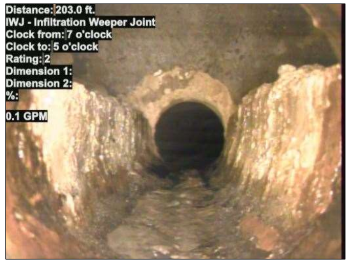
Photo: 15_029-15_030-20230724-164719.JPG At: 203 ft. 7/5 IWJ - Infiltration Weeper Joint Joint: Yes 0.1 GPM
