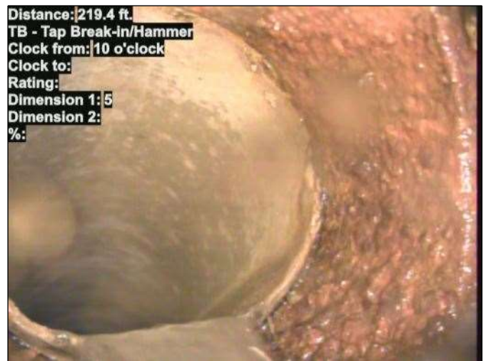
Photo: 15_048-15_033-20230725-104545.JPG At: 219.4 ft. 10/. TB - Tap Break-in/Hammer Joint: No
