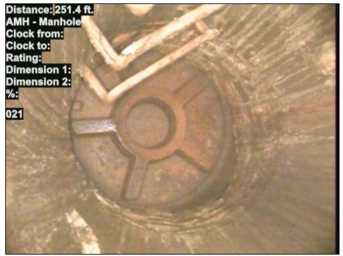
Photo: 15_020-15_021-20230724-153207.JPG At: 251.4 ft. AMH - Manhole Joint: No 021
