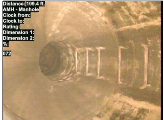
Photo: 15_071-15_072-20230726-082516.JPG At: 109.4 ft. AMH - Manhole Joint: No 072
