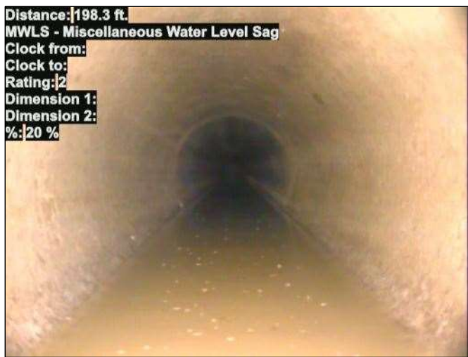
Photo: 15_035-15_034-20230801-085320.JPG At: 198.3 ft. MWLS - Miscellaneous Water Level Sag Joint: No 20 %
