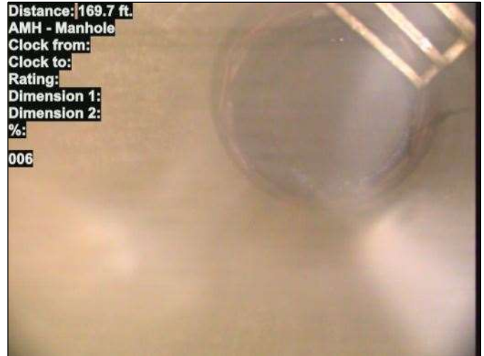
Photo: 15_007-15_006-20230726-125310.JPG At: 169.7 ft. AMH - Manhole Joint: No 006
