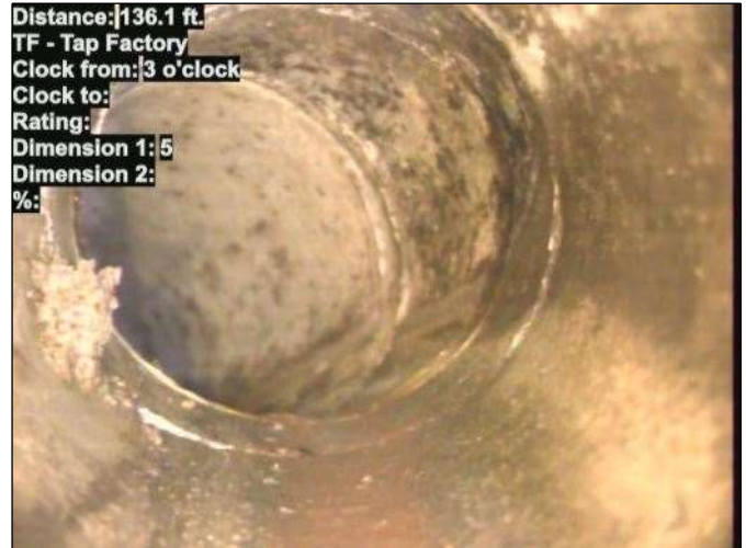
Photo: 15_028-15_029-20230724-163421.JPG At: 136.1 ft. 3/. TF - Tap Factory Joint: No
