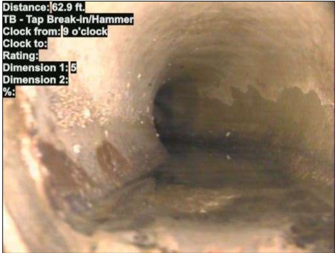
Photo: 15_009-15_009A-20230726-103622.JPG At: 62.9 ft. 9/. TB - Tap Break-in/Hammer Joint: No
