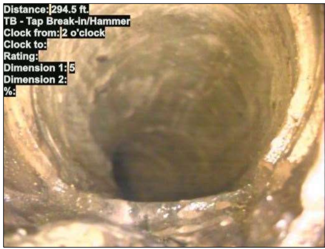
Photo: 15_014-15_015-20230724-144716.JPG At: 294.5 ft. 2/. TB - Tap Break-in/Hammer Joint: No
