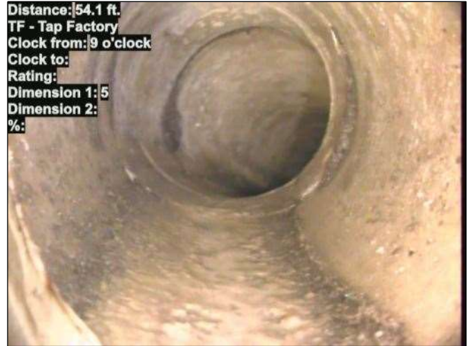
Photo: 15_027-15_026-20230725-182640.JPG At: 54.1 ft. 9/. TF - Tap Factory Joint: No
