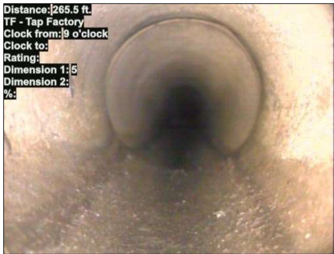
Photo: 15_077-15_078-20230801-072316.JPG At: 265.5 ft. 9/. TF - Tap Factory Joint: No
