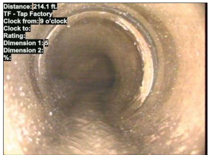
Photo: 15_042-15_043-20230801-131209.JPG At: 214.1 ft. 9/. TF - Tap Factory Joint: No
