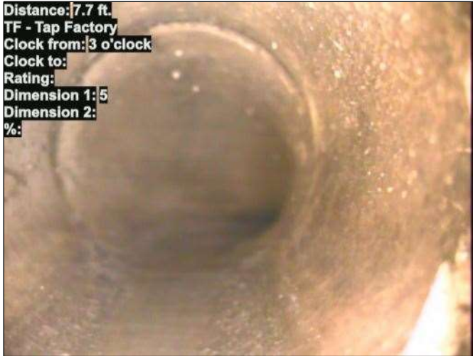
Photo: 15_080-15_079-20230801-080437.JPG At: 7.7 ft. 3/. TF - Tap Factory Joint: No
