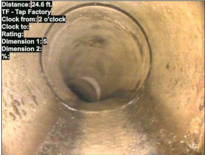
Photo: 15_057-15_046-20230725-080904.JPG At: 24.6 ft. 2/. TF - Tap Factory Joint: No
