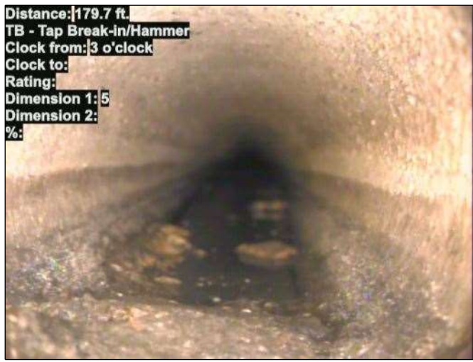
Photo: 15_077-15_078-20230801-072022.JPG At: 179.7 ft. 3/. TB - Tap Break-in/Hammer Joint: No
