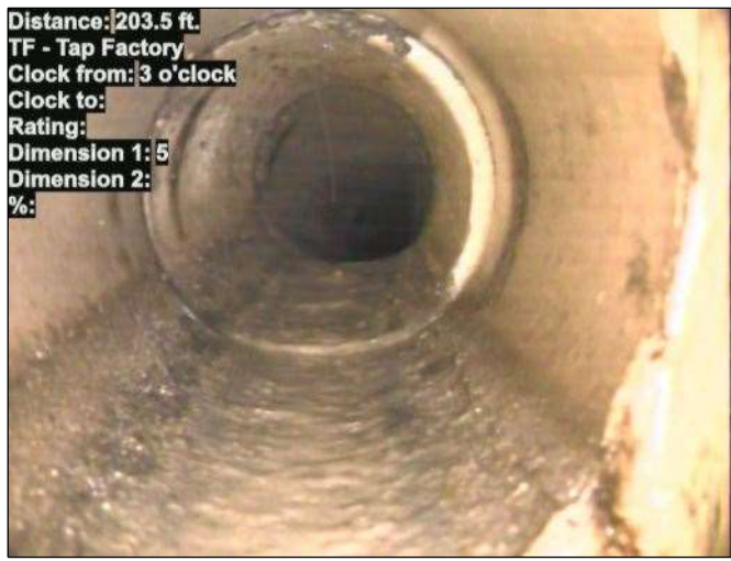
Photo: 15_027-15_026-20230725-183326.JPG At: 203.5 ft. 3/. TF - Tap Factory Joint: No
