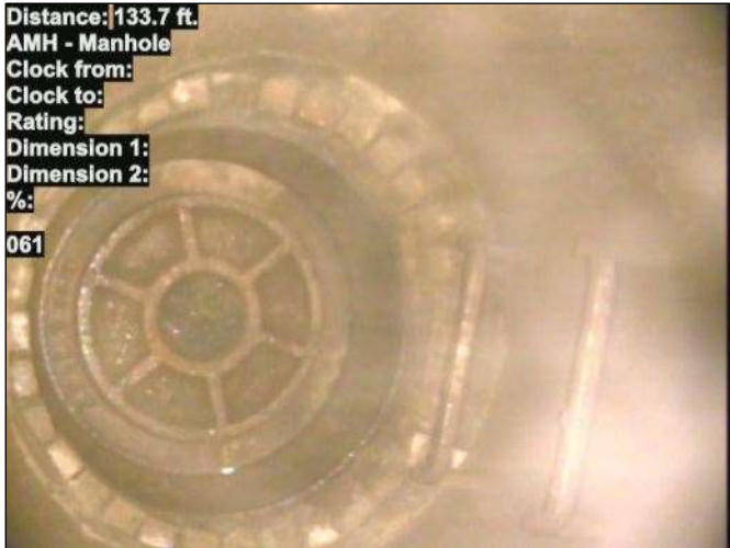
Photo: 15_078-15_061-20230801-082420.JPG At: 133.7 ft. AMH - Manhole Joint: No 061
