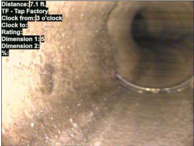
Photo: 15_056-15_057-20230725-074305.JPG At: 7.1 ft. 3/. TF - Tap Factory Joint: No
