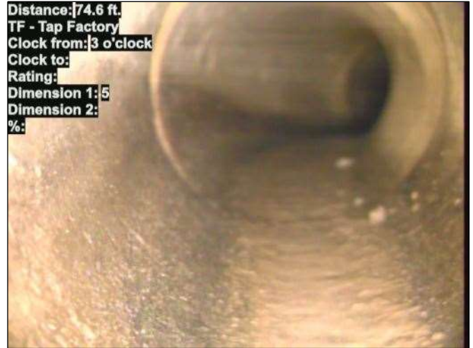
Photo: 15_037-15_038-20230724-121936.JPG At: 74.6 ft. 3/. TF - Tap Factory Joint: No
