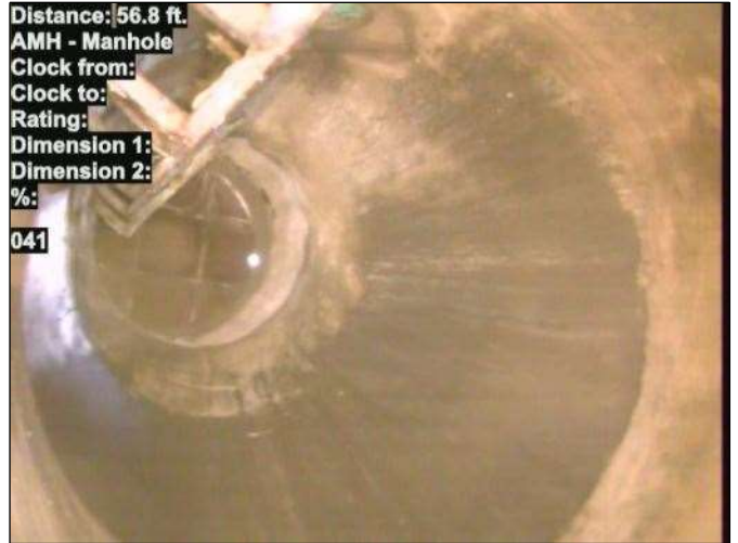
Photo: 15_040-15_041-20230801-123328.JPG At: 56.8 ft. AMH - Manhole Joint: No 041
