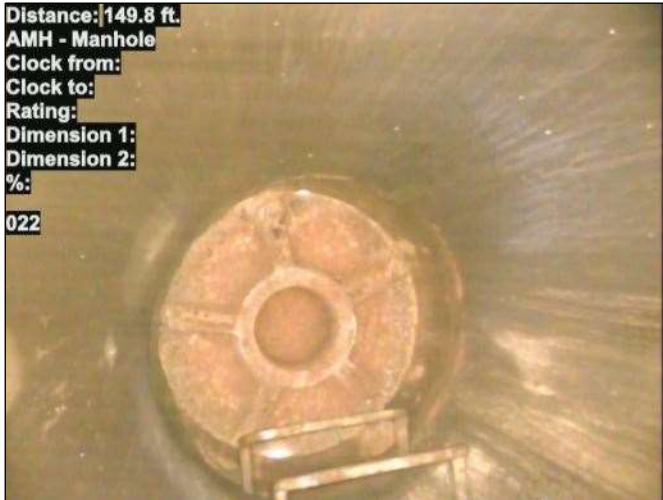
Photo: 15_021-15_022-20230724-153957.JPG At: 149.8 ft. AMH - Manhole Joint: No 022
