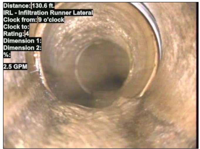
Photo: 15_022-15_023-20230724-154903.JPG At: 130.6 ft. 9/. IRL - Infiltration Runner Lateral Joint: No 2.5 GPM
