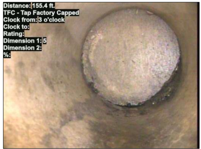
Photo: 15_035-15_034-20230801-085143.JPG At: 155.4 ft. 3/. TFC - Tap Factory Capped Joint: No
