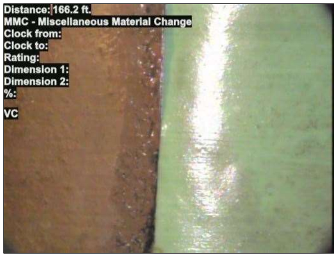
Photo: 15_005-15_018-20230801-092022.JPG At: 166.2 ft. MMC - Miscellaneous Material Change Joint: No VC
