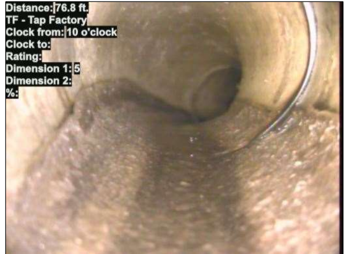
Photo: 15_029-15_030-20230724-164331.JPG At: 76.8 ft. 10/. TF - Tap Factory Joint: No
