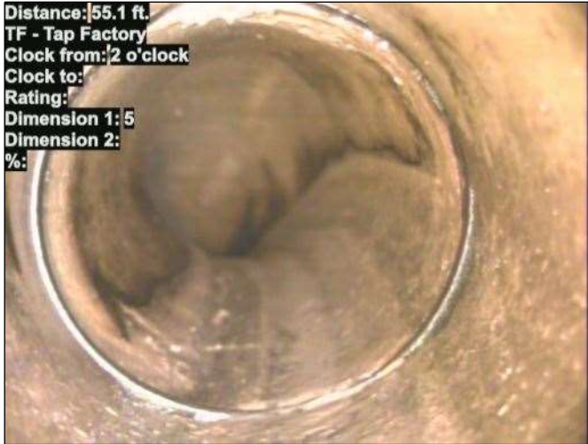
Photo: 15_017-15_018-20230724-150507.JPG At: 55.1 ft. 2/. TF - Tap Factory Joint: No
