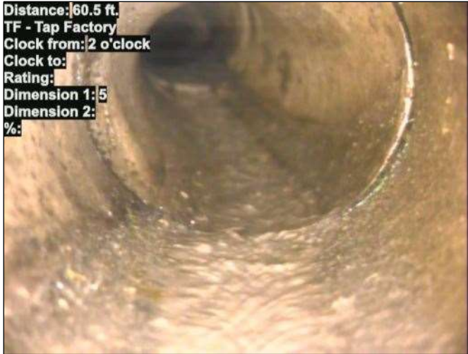
Photo: 15_029-15_030-20230724-164204.JPG At: 60.5 ft. 2/. TF - Tap Factory Joint: No
