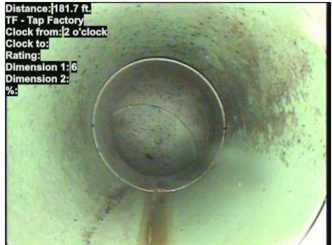
Photo: 15_058-15_059-20230804-073627.JPG At: 181.7 ft. 2/. TF - Tap Factory Joint: No
