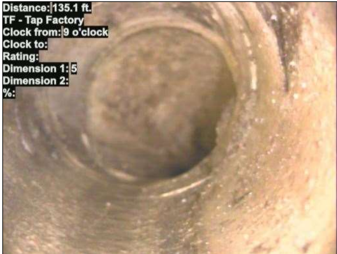
Photo: 15_028-15_029-20230724-163402.JPG At: 135.1 ft. 9/. TF - Tap Factory Joint: No
