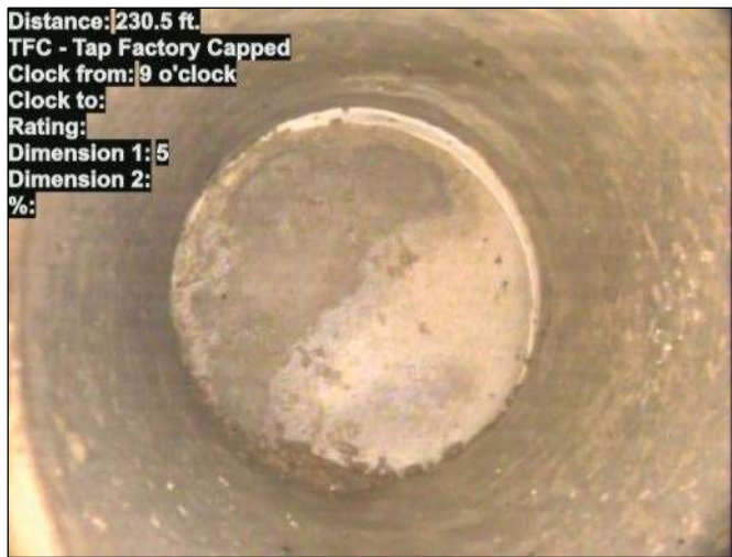
Photo: 15_027-15_026-20230725-183456.JPG At: 230.5 ft. 9/. TFC - Tap Factory Capped Joint: No
