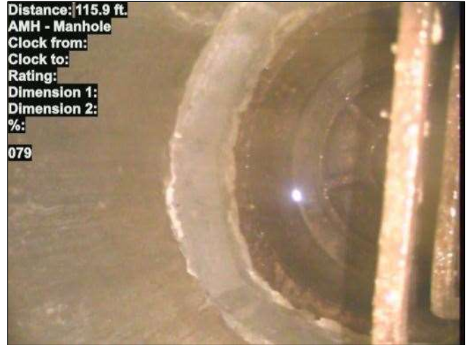
Photo: 15_080-15_079-20230801-080815.JPG At: 115.9 ft. AMH - Manhole Joint: No 079
