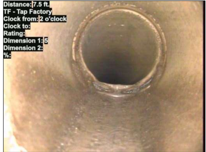
Photo: STUB-15_070-20230726-094417.JPG At: 7.5 ft. 2/. TF - Tap Factory Joint: No
