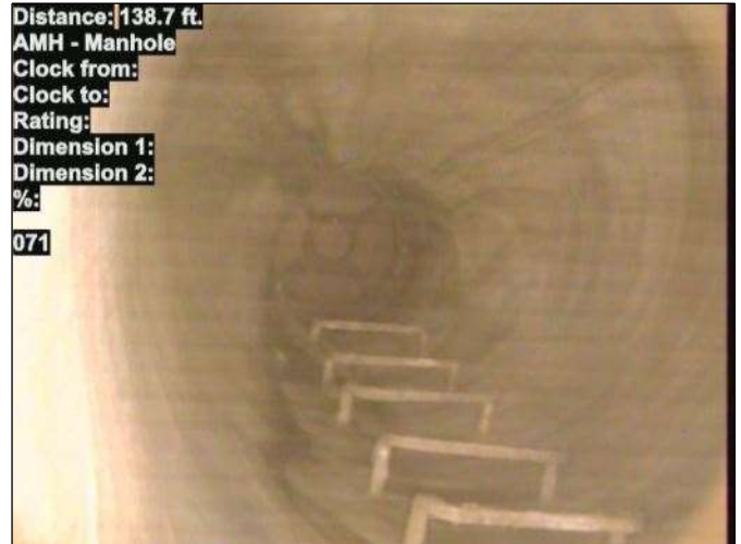
Photo: 15_070-15_071-20230726-081636.JPG At: 138.7 ft. AMH - Manhole Joint: No 071
