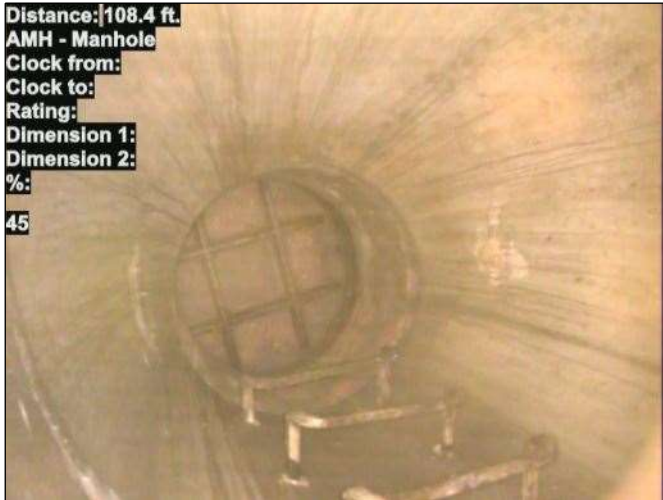
Photo: 15_044-15_045-20230725-085837.JPG At: 108.4 ft. AMH - Manhole Joint: No 45
