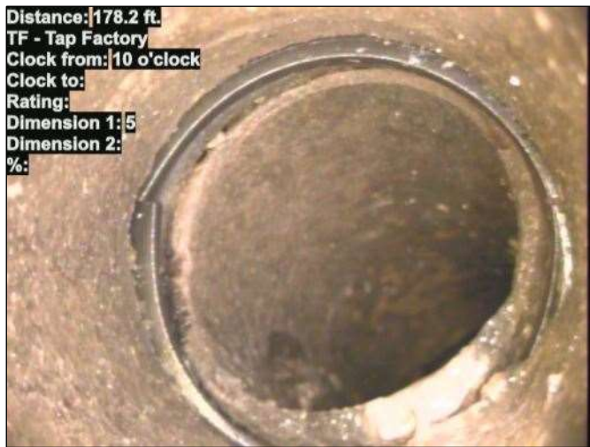
Distance: 178.2 ft. TF - Tap Factory Clock from: 10 o'clock Clock to: Rating: Dimension 1: 5 Dimension 2: %: Photo: 15_014-15_015-20230724-144249.JPG At: 178.2 ft. 10/. TF - Tap Factory Joint: No
