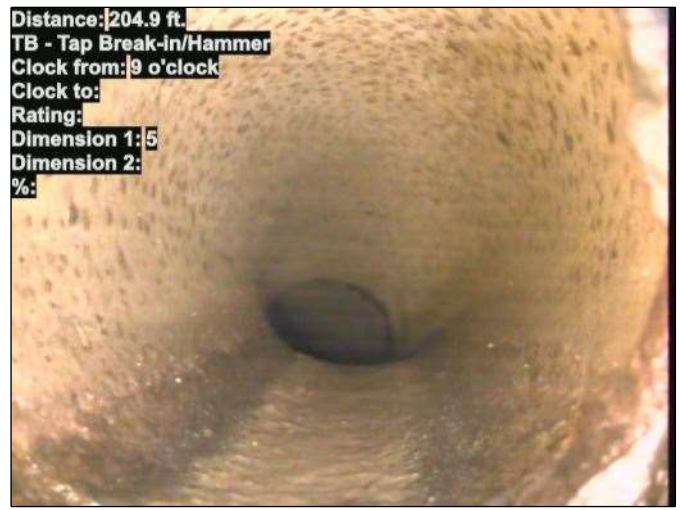
Photo: 15_027-15_026-20230725-183345.JPG At: 204.9 ft. 9/. TB - Tap Break-in/Hammer Joint: No
