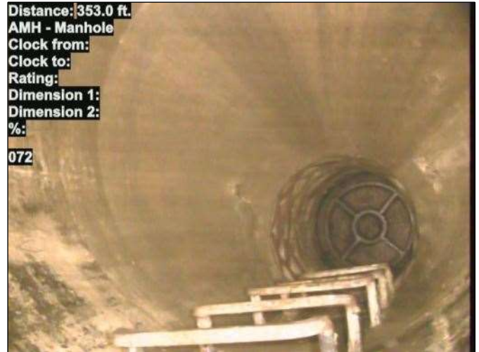
Photo: 15_073-15_072-20230726-074332.JPG At: 353 ft. AMH - Manhole Joint: No 072
