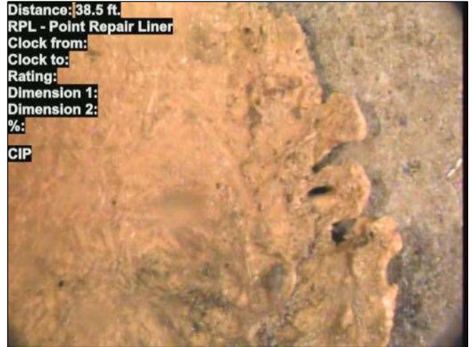
Photo: 15_025-15_024-20230801-095934.JPG At: 38.5 ft. RPL - Point Repair Liner Joint: No CIP
