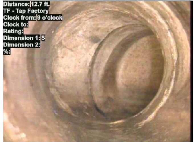
Photo: 15_031-15_032-20230724-165851.JPG At: 12.7 ft. 9/. TF - Tap Factory Joint: No
