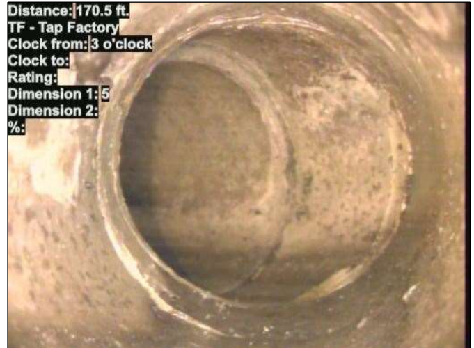
Photo: 15_031-15_032-20230724-170347.JPG At: 170.5 ft. 3/. TF - Tap Factory Joint: No
