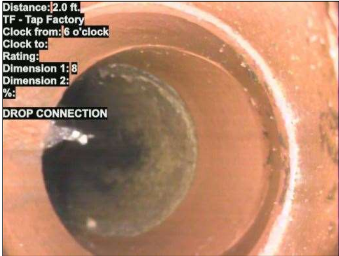
Photo: 15_048-15_033-20230725-103219.JPG At: 2 ft. 6/. TF - Tap Factory Joint: No DROP CONNECTION
