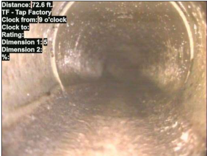
Photo: 15_030-15_031-20230724-165404.JPG At: 72.6 ft. 9/. TF - Tap Factory Joint: No
