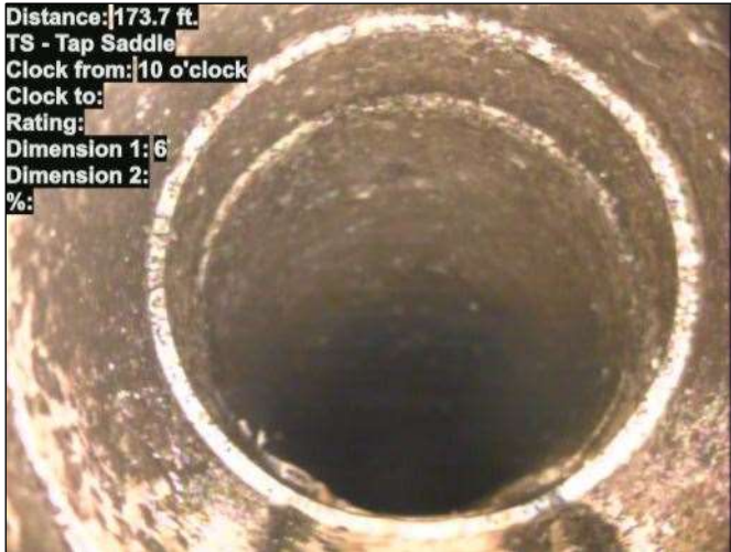
Photo: 15_038-15_039-20230724-123759.JPG At: 173.7 ft. 10/. TS - Tap Saddle Joint: No
