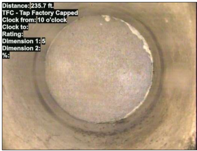
Photo: 15_048-15_033-20230725-104634.JPG At: 235.7 ft. 10/. TFC - Tap Factory Capped Joint: No
