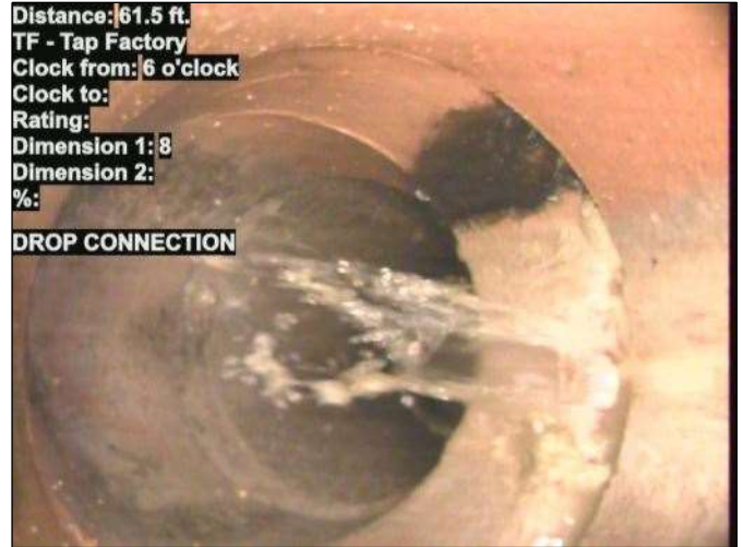
Photo: 15_032-15_033-20230725-071722.JPG At: 61.5 ft. 6/. TF - Tap Factory Joint: No DROP CONNECTION
