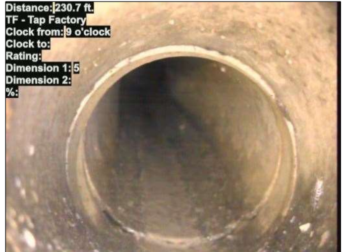
Photo: 15_038-15_039-20230724-123945.JPG At: 230.7 ft. 9/. TF - Tap Factory Joint: No
