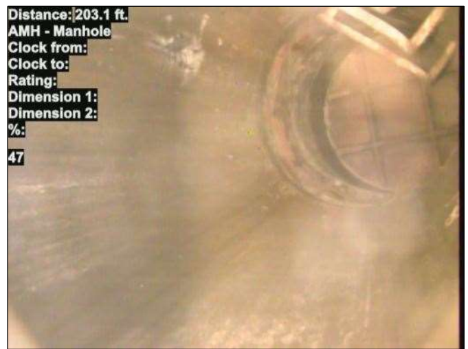
Photo: 15_046-15_047-20230725-092939.JPG At: 203.1 ft. AMH - Manhole Joint: No 47
