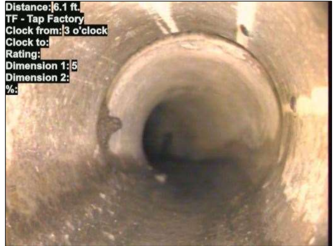
Photo: STUB-15_013-20230725-130206.JPG At: 6.1 ft. 3/. TF - Tap Factory Joint: No
