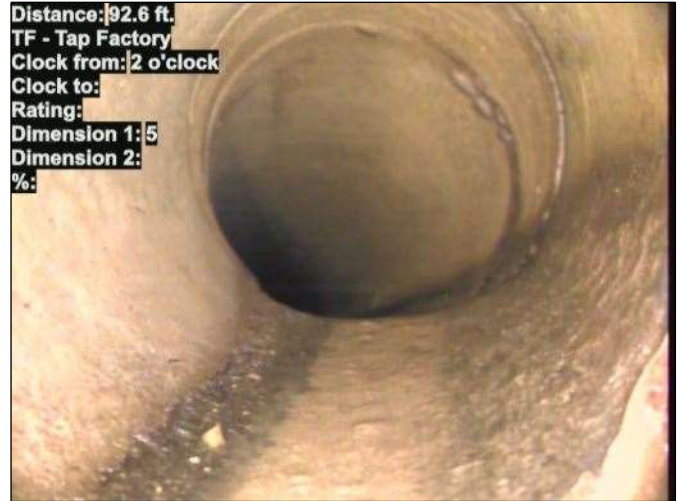
Photo: 15_050-15_051-20230726-070701.JPG At: 92.6 ft. 2/. TF - Tap Factory Joint: No
