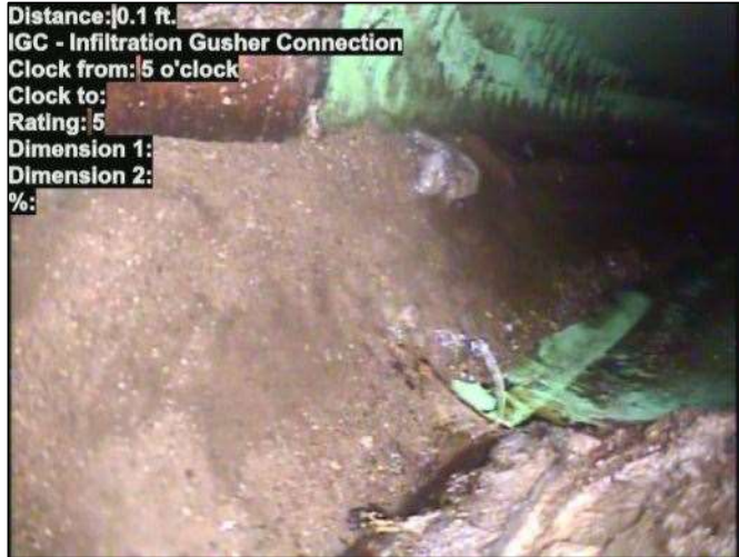
Photo: 15_115-15_003-20230804-132528.JPG At: 0.1 ft. 5/. IGC - Infiltration Gusher Connection Joint: No
