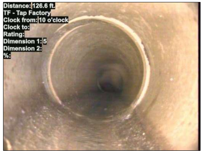
Photo: 15_046-15_047-20230725-092633.JPG At: 126.6 ft. 10/. TF - Tap Factory Joint: No
