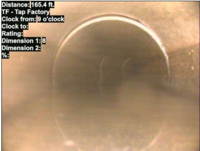
Photo: 15_007-15_006-20230726-125145.JPG At: 165.4 ft. 9/. TF - Tap Factory Joint: No
