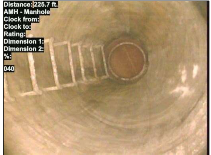
Photo: 15_036-15_040-20230801-112235.JPG At: 225.7 ft. AMH - Manhole Joint: No 040
