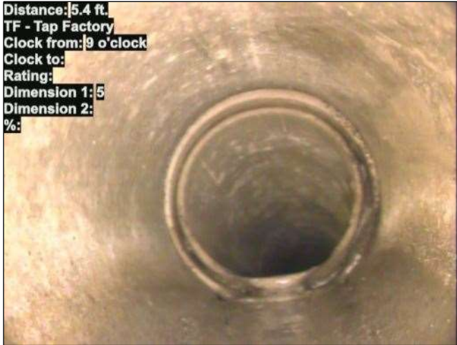
Photo: STUB-15_070-20230726-094356.JPG At: 5.4 ft. 9/. TF - Tap Factory Joint: No
