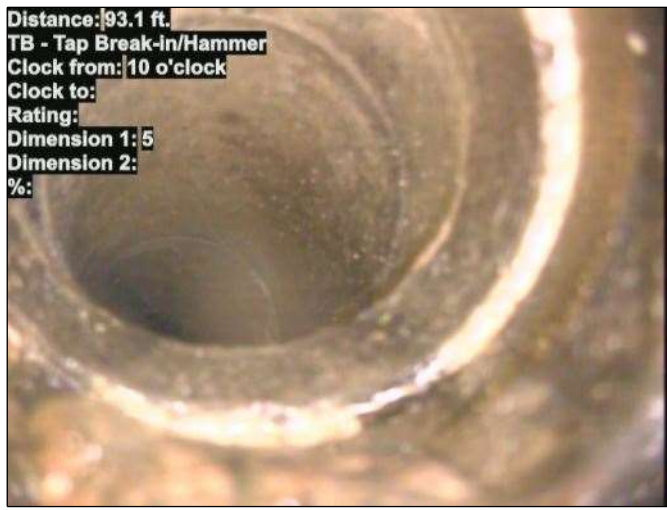
Photo: 15_025-15_024-20230801-100247.JPG At: 93.1 ft. 10/. TB - Tap Break-in/Hammer Joint: No
