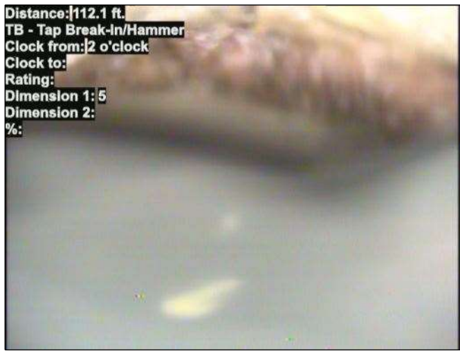
Photo: 15_062-15_081-20230804-122810.JPG At: 112.1 ft. 2/. TB - Tap Break-in/Hammer Joint: No
