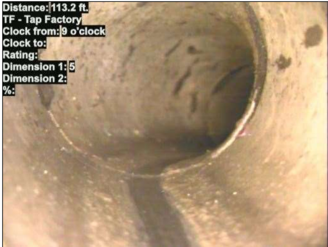
Photo: 15_020-15_021-20230724-152641.JPG At: 113.2 ft. 9/. TF - Tap Factory Joint: No
