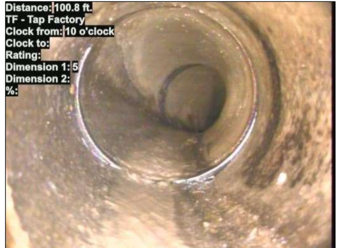
Photo: 15_035-15_034-20230801-084822.JPG At: 100.8 ft. 10/. TF - Tap Factory Joint: No
