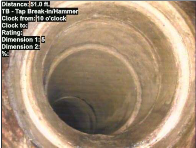
Photo: 15_026-15_024-20230725-184620.JPG At: 51 ft. 10/. TB - Tap Break-in/Hammer Joint: No
