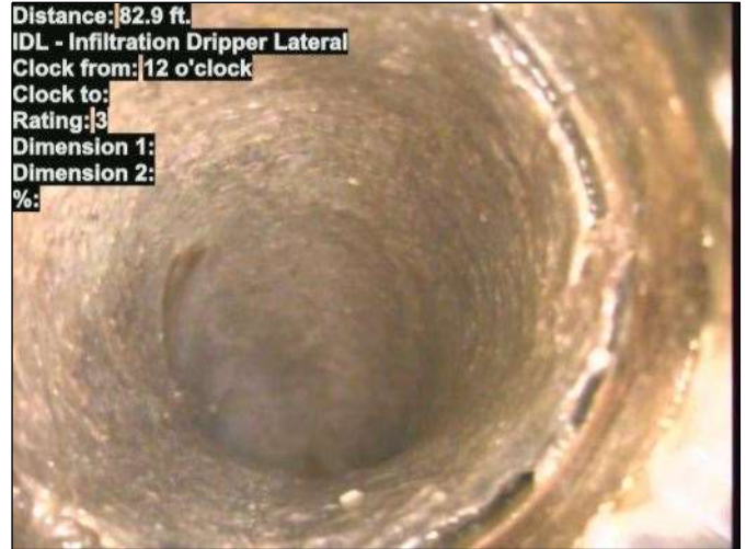
Photo: 15_033-15_034-20230801-104544.JPG At: 82.9 ft. 12/. IDL - Infiltration Dripper Lateral Joint: No
