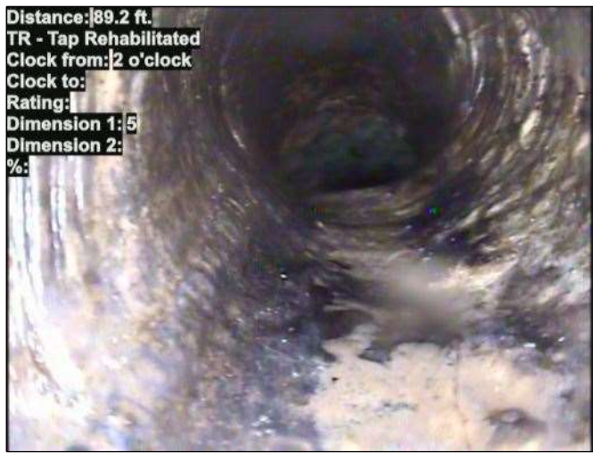
Photo: 15_043-15_058-20230804-072107.JPG At: 89.2 ft. 2/. TR - Tap Rehabilitated Joint: No
