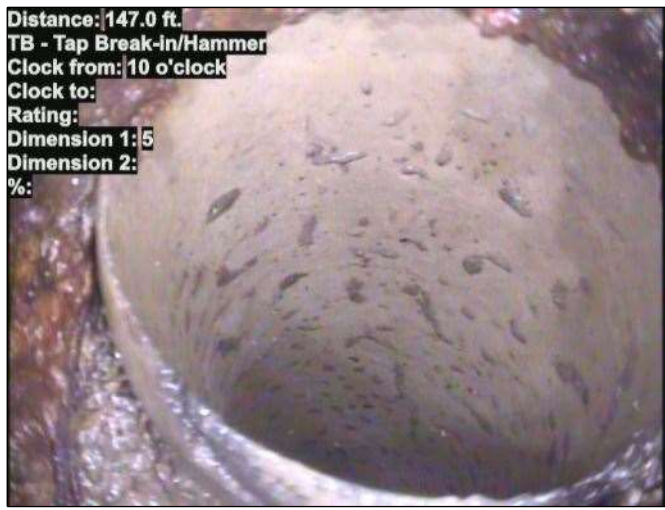
Photo: 15_092-15_062-20230804-112744.JPG At: 147 ft. 10/. TB - Tap Break-in/Hammer Joint: No
