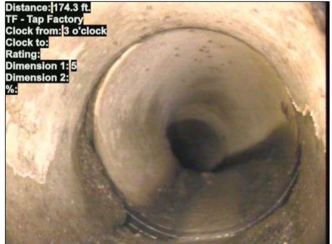
Photo: 15_037-15_038-20230724-122316.JPG At: 174.3 ft. 3/. TF - Tap Factory Joint: No
