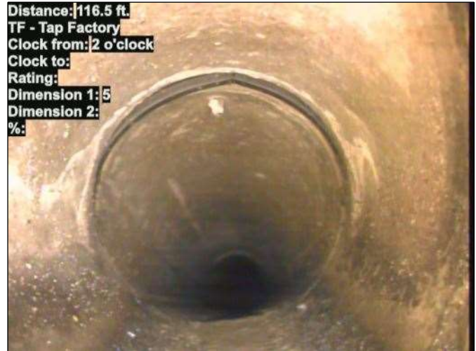
Photo: 15_056-15_057-20230725-074708.JPG At: 116.5 ft. 2/. TF - Tap Factory Joint: No
