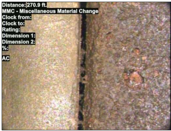
Photo: 15_001-15_002-20230725-122611.JPG At: 270.9 ft. MMC - Miscellaneous Material Change Joint: No AC
