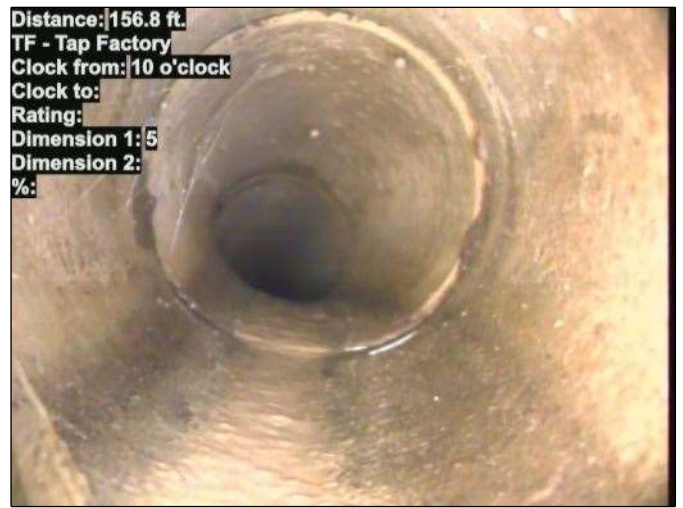
Distance: 156.8 ft. TF - Tap Factory Clock from: 10 o'clock Clock to: Rating: 5 Dimension 1: 5 Dimension 2: %: Photo: 15_019-15_018-20230721-114812.JPG At: 156.8 ft. 10/. TF - Tap Factory Joint: No
