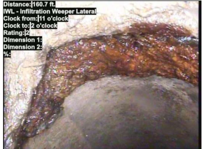
Photo: 15_058-15_059-20230804-073521.JPG At: 160.7 ft. IWL - Infiltration Weeper Lateral 11/2 Joint: No
