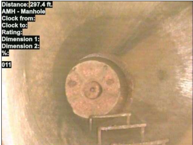
Photo: 15_012-15_011-20230726-101942.JPG At: 297.4 ft. AMH - Manhole Joint: No 011
