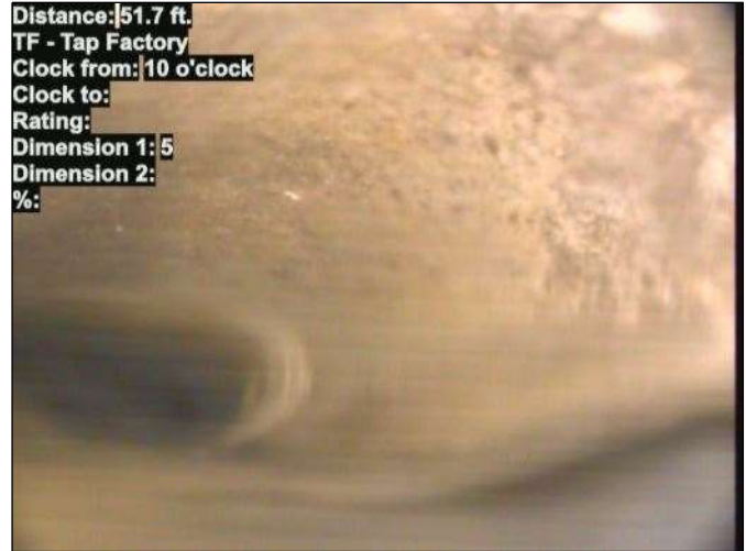
Photo: 15_041-15_042-20230801-124003.JPG At: 51.7 ft. 10/. TF - Tap Factory Joint: No
