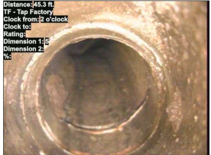
Photo: 15_030-15_031-20230724-165253.JPG At: 45.3 ft. 2/. TF - Tap Factory Joint: No
