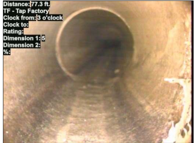
Photo: 15_074-15_075-20230726-084338.JPG At: 77.3 ft. 3/. TF - Tap Factory Joint: No
