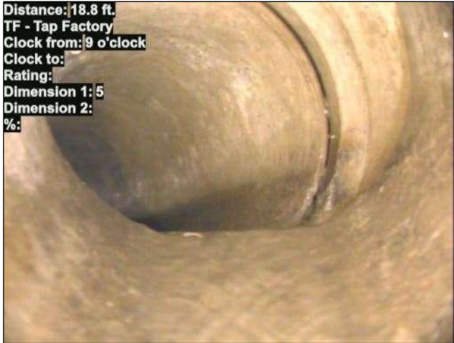
Photo: 15_014-15_015-20230724-143457.JPG At: 18.8 ft. 9/. TF - Tap Factory Joint: No
