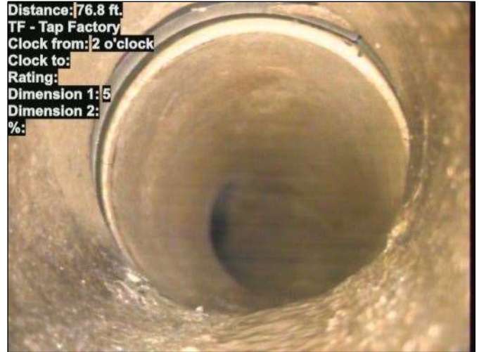
Photo: 15_023-15_024-20230724-155643.JPG At: 76.8 ft. 2/. TF - Tap Factory Joint: No
