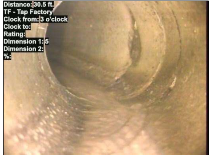
Photo: 15_028-15_029-20230724-163112.JPG At: 30.5 ft. 3/. TF - Tap Factory Joint: No
