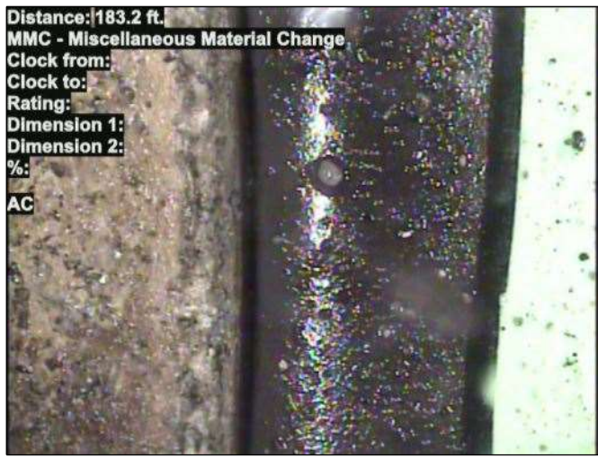
Photo: 15_058-15_059-20230804-073642.JPG At: 183.2 ft. MMC - Miscellaneous Material Change Joint: No AC
