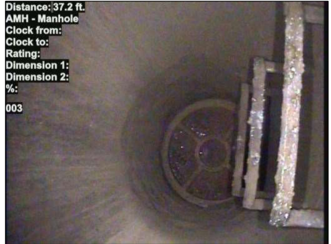
Photo: 15_115-15_003-20230804-132429.JPG At: 37.2 ft. AMH - Manhole Joint: No 003
