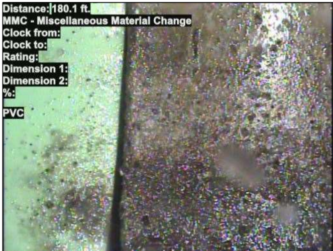
Photo: 15_058-15_059-20230804-073611.JPG At: 180.1 ft. MMC - Miscellaneous Material Change Joint: No PVC
