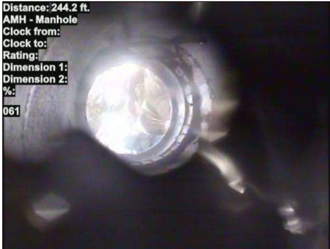
Photo: 15_060-15_061-20230804-102229.JPG At: 244.2 ft. AMH - Manhole Joint: No 061
