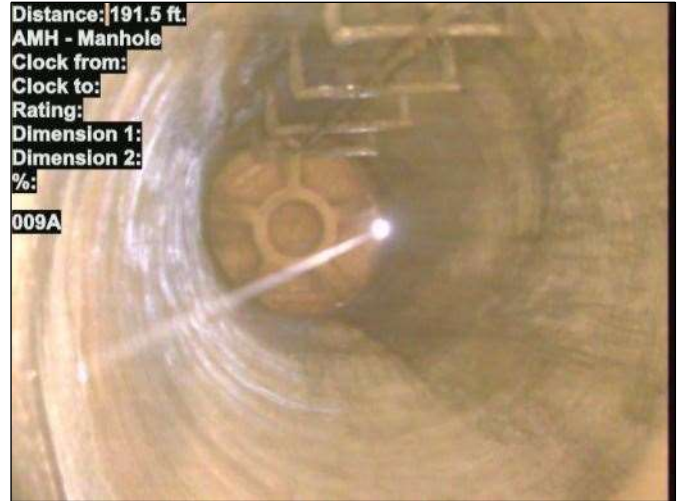
Photo: 15_009-15_009A-20230726-104100.JPG At: 191.5 ft. AMH - Manhole Joint: No 009A
