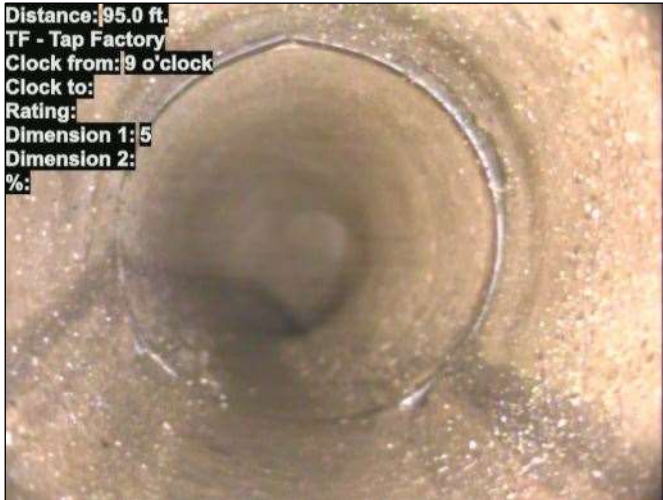
Photo: 15_042-15_043-20230801-130600.JPG At: 95 ft. 9/. TF - Tap Factory Joint: No
