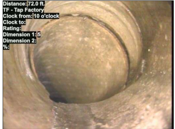
Photo: 15_014-15_015-20230724-143650.JPG At: 72 ft. 10/. TF - Tap Factory Joint: No
