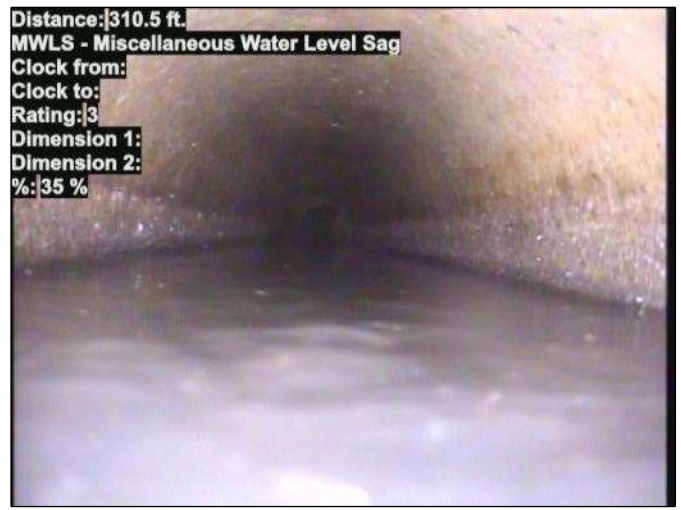
Photo: 15_058-15_059-20230804-074004.JPG At: 310.5 ft. MWLS - Miscellaneous Water Level Sag Joint: No 35 %
