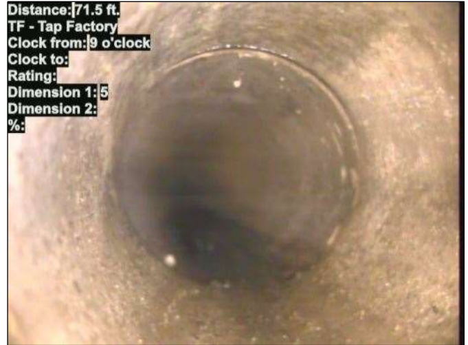
Photo: 15_079-15_078-20230801-081627.JPG At: 71.5 ft. 9/. TF - Tap Factory Joint: No
