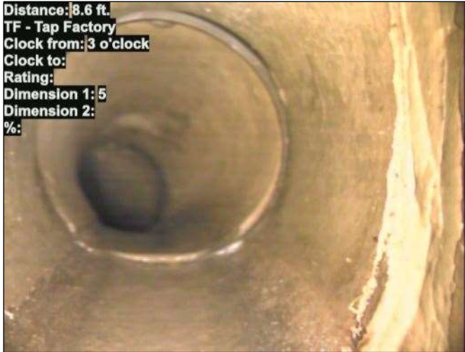
Photo: 15_049-15_050-20230726-063524.JPG At: 8.6 ft. 3/. TF - Tap Factory Joint: No
