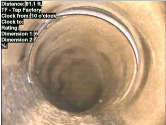
Photo: 15_023-15_024-20230724-155732.JPG At: 91.1 ft. 10/. TF - Tap Factory Joint: No
