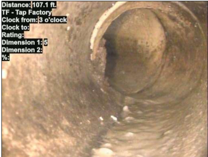
Photo: 15_027-15_026-20230725-182849.JPG At: 107.1 ft. 3/. TF - Tap Factory Joint: No
