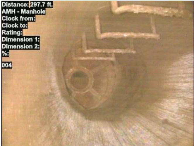
Photo: 15_003-15_004-20230725-114559.JPG At: 297.7 ft. AMH - Manhole Joint: No 004
