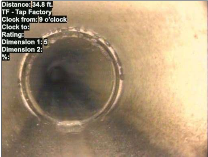
Photo: 15_074-15_075-20230726-084200.JPG At: 34.8 ft. 9/. TF - Tap Factory Joint: No
