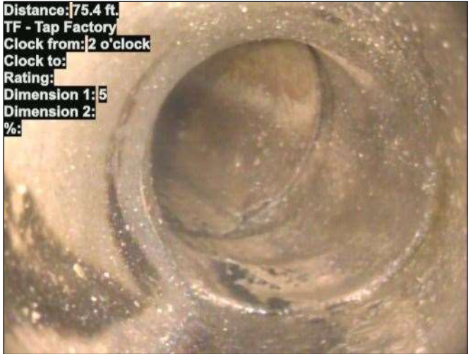
Photo: 15_024-15_033-20230801-101123.JPG At: 75.4 ft. 2/. TF - Tap Factory Joint: No
