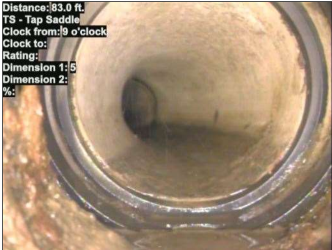
Photo: 15_019-15_018-20230721-114440.JPG At: 83 ft. 9/. TS - Tap Saddle Joint: No
