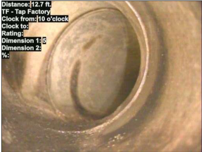
Photo: 15_035-15_034-20230801-084300.JPG At: 12.7 ft. 10/. TF - Tap Factory Joint: No
