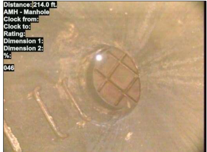
Photo: 15_057-15_046-20230725-081624.JPG At: 214 ft. AMH - Manhole Joint: No 046
