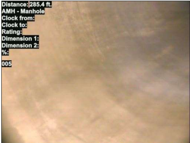
Photo: 15_004-15_005-20230725-120135.JPG At: 285.4 ft. AMH - Manhole Joint: No 005
