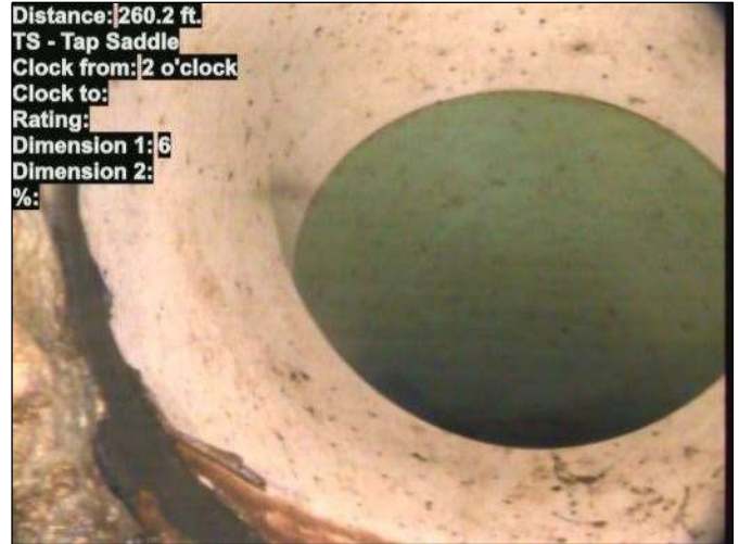
Photo: 15_003-15_004-20230725-114418.JPG At: 260.2 ft. 2/. TS - Tap Saddle Joint: No
