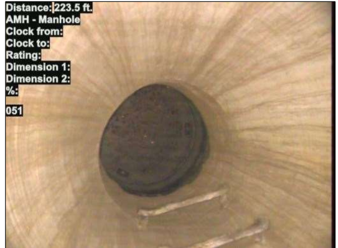
Photo: 15_050-15_051-20230726-071208.JPG At: 223.5 ft. AMH - Manhole Joint: No 051
