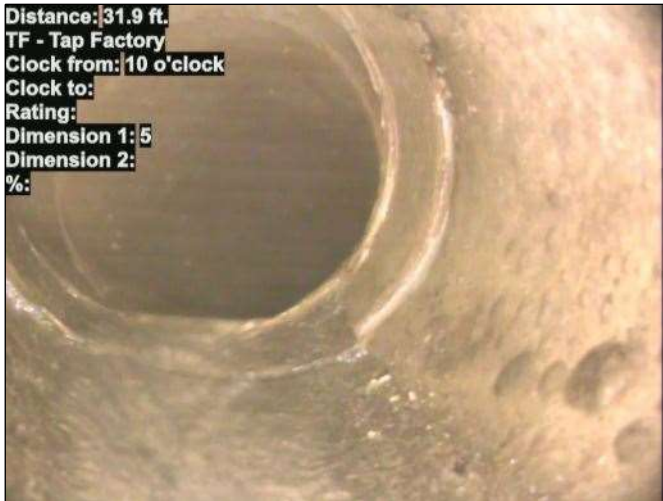
Photo: 15_039-15_040-20230724-124329.JPG At: 31.9 ft. 10/. TF - Tap Factory Joint: No
