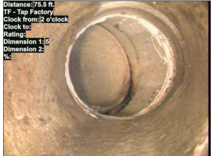
Photo: 15_019-15_018-20230721-114359.JPG At: 75.5 ft. 2/. TF - Tap Factory Joint: No
