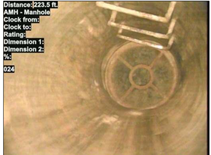
Photo: 15_023-15_024-20230724-160303.JPG At: 223.5 ft. AMH - Manhole Joint: No 024
