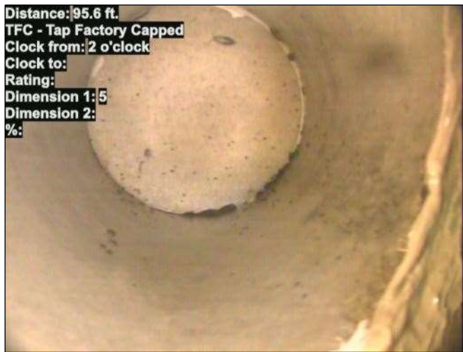
Distance: 95.6 ft. TFC - Tap Factory Capped Clock from: 2 o'clock Clock to: Rating: Dimension 1: 5 Dimension 2: %: Photo: 15_045-15_046-20230725-091102.JPG At: 95.6 ft. 2/. TFC - Tap Factory Capped Joint: No
