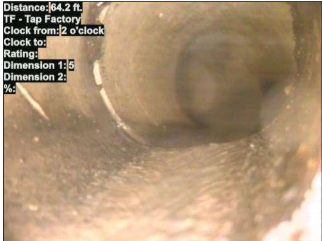
Photo: 15_022-15_023-20230724-154609.JPG At: 64.2 ft. 2/ TF - Tap Factory Joint: No
