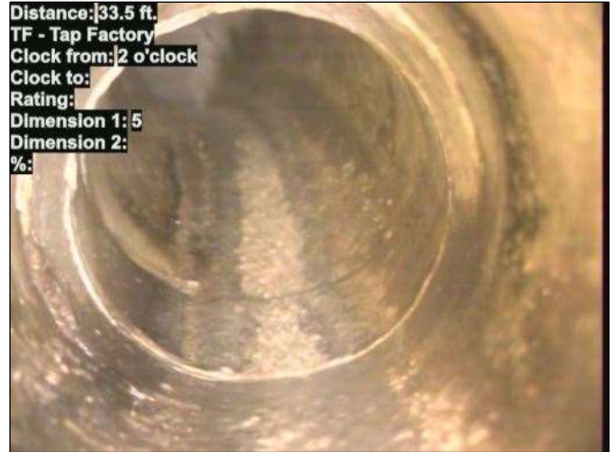
Photo: 15_035-15_034-20230801-084358.JPG At: 33.5 ft. 2/. TF - Tap Factory Joint: No
