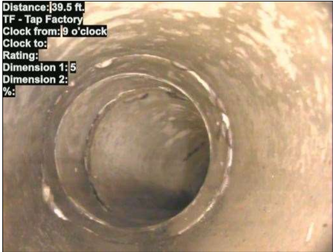
Photo: 15_050-15_051-20230726-070443.JPG At: 39.5 ft. 9/. TF - Tap Factory Joint: No
