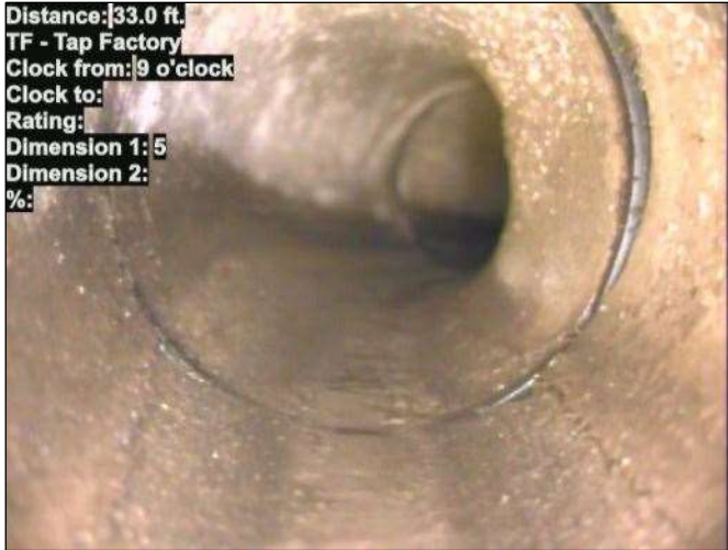
Photo: 15_020-15_021-20230724-152349.JPG At: 33 ft. 9/. TF - Tap Factory Joint: No
