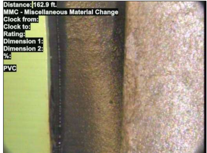
Photo: 15_005-15_018-20230801-091958.JPG At: 162.9 ft. MMC - Miscellaneous Material Change Joint: No PVC
