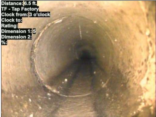
Photo: 15_019-15_018-20230721-114038.JPG At: 6.5 ft. 3/. TF - Tap Factory Joint: No
