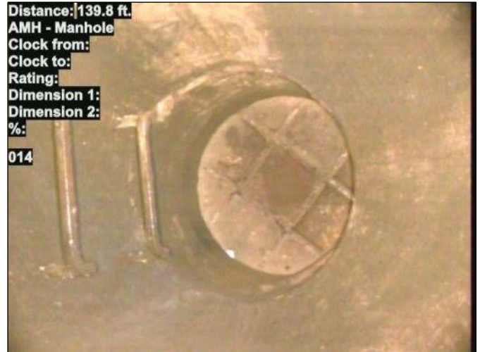
Photo: 15_013-15_014-20230725-125220.JPG At: 139.8 ft. AMH - Manhole Joint: No 014
