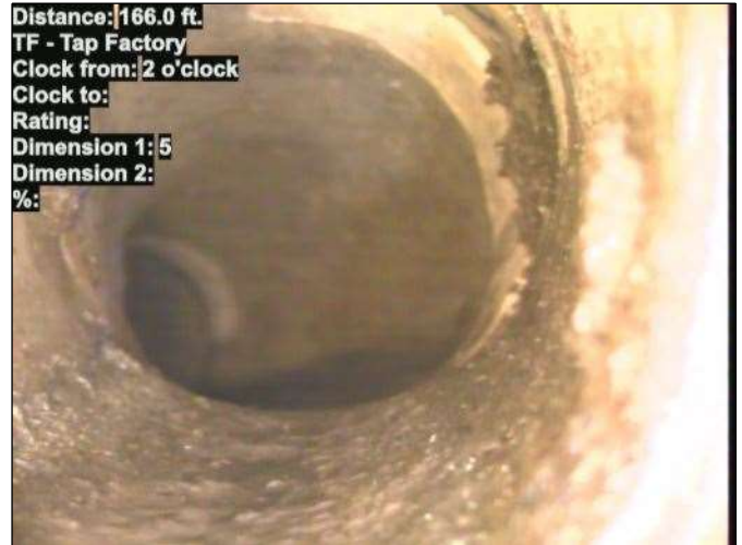
Photo: 15_020-15_021-20230724-152826.JPG At: 166 ft. 2/. TF - Tap Factory Joint: No
