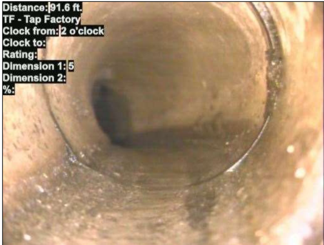
Photo: 15_031-15_032-20230724-170120.JPG At: 91.6 ft. 2/. TF - Tap Factory Joint: No
