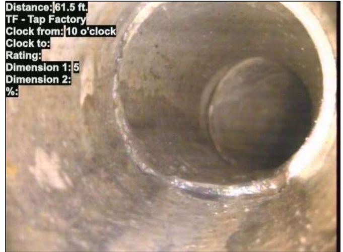
Photo: 15_029-15_030-20230724-164223.JPG At: 61.5 ft. 10/. TF - Tap Factory Joint: No
