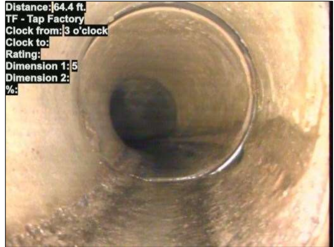
Photo: 15_057-15_046-20230725-081046.JPG At: 64.4 ft. 3/. TF - Tap Factory Joint: No
