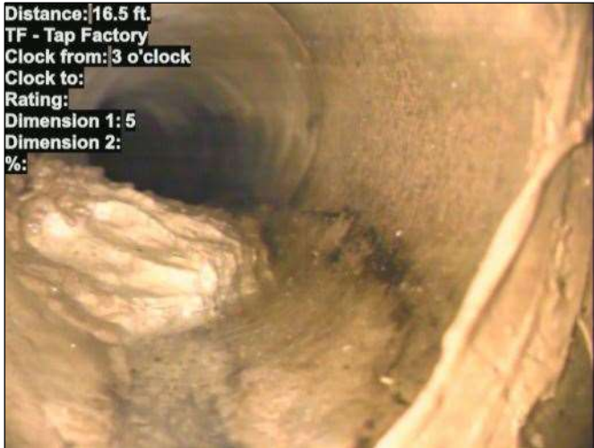
Photo: 15_077-15_078-20230801-071511.JPG At: 16.5 ft. 3/. TF - Tap Factory Joint: No
