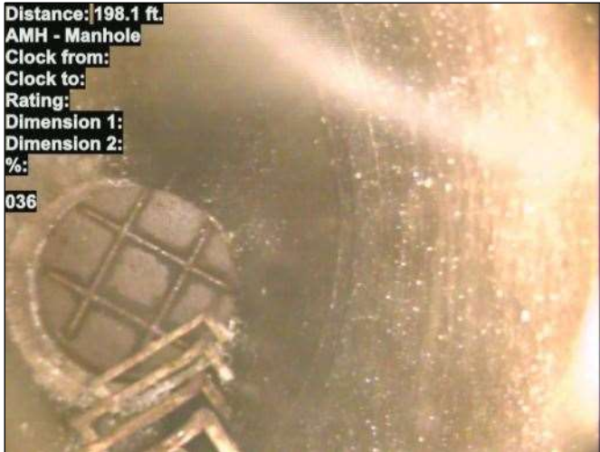
Photo: 15_034-15_036-20230801-110135.JPG At: 198.1 ft. AMH - Manhole Joint: No 036
