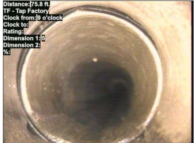
Photo: 15_021-15_022-20230724-153703.JPG At: 75.8 ft. 9/. TF - Tap Factory Joint: No
