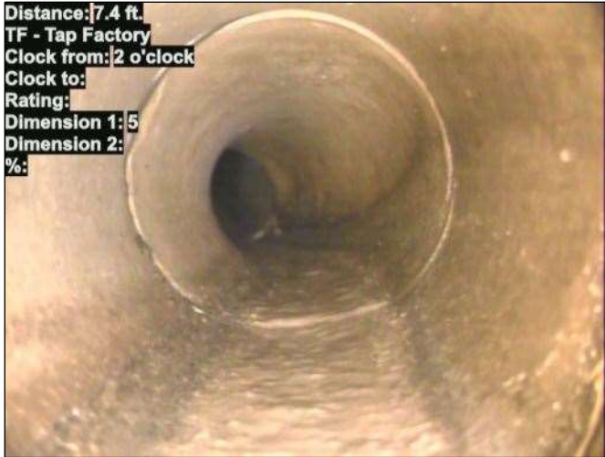
Photo: 15_045-15_046-20230725-090238.JPG At: 7.4 ft. 2/. TF - Tap Factory Joint: No
