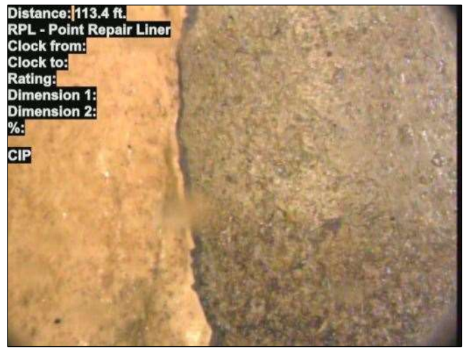
Photo: 15_025-15_024-20230801-100340.JPG At: 113.4 ft. RPL - Point Repair Liner Joint: No CIP
