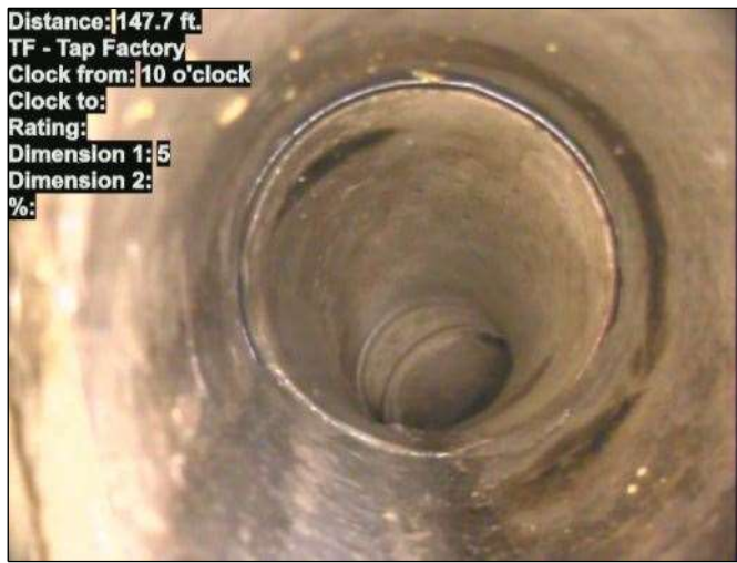
Photo: 15_035-15_034-20230801-085109.JPG At: 147.7 ft. 10/. TF - Tap Factory Joint: No
