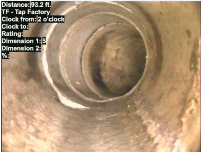
Photo: 15_035-15_034-20230801-084730.JPG At: 93.2 ft. 2/. TF - Tap Factory Joint: No
