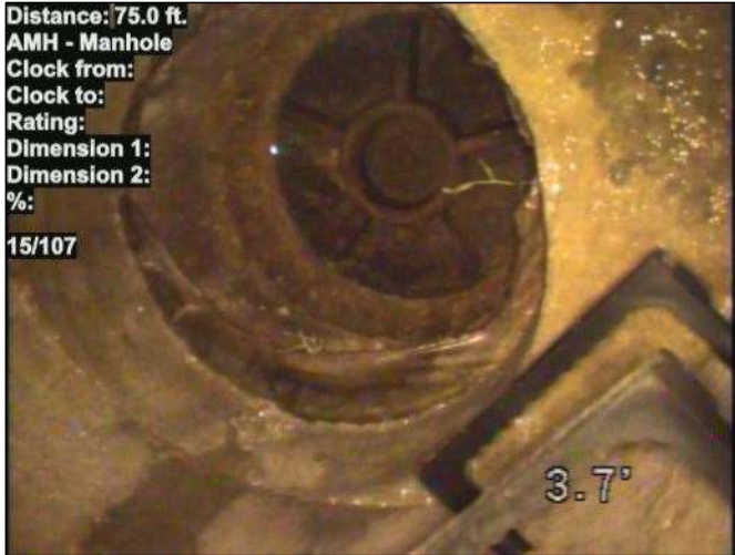
Photo: 15_107-15_110-20230807-101503.JPG At: 75 ft. AMH - Manhole Joint: No 15/107
