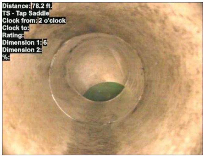
Photo: 15_029-15_030-20230724-164402.JPG At: 78.2 ft. 2/ TS - Tap Saddle Joint: No
