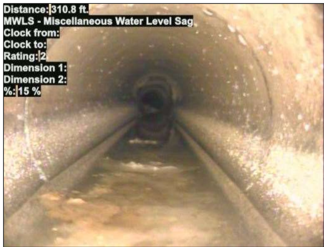
Photo: 15_037-15_038-20230724-122952.JPG At: 310.8 ft. MWLS - Miscellaneous Water Level Sag Joint: No 15 %
