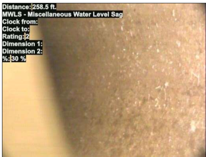
Photo: 15_042-15_043-20230801-131503.JPG At: 258.5 ft. MWLS - Miscellaneous Water Level Sag Joint: No 30 %
