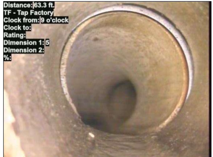
Photo: 15_022-15_023-20230724-154553.JPG At: 63.3 ft. 9/ TF - Tap Factory Joint: No
