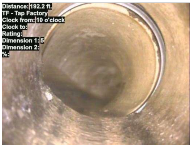
Photo: 15_022-15_023-20230724-155121.JPG At: 192.2 ft. 10/. TF - Tap Factory Joint: No
