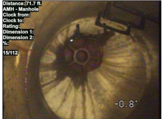
Photo: 15_111-15_112-20230807-102505.JPG At: 71.7 ft. AMH - Manhole Joint: No 15/112
