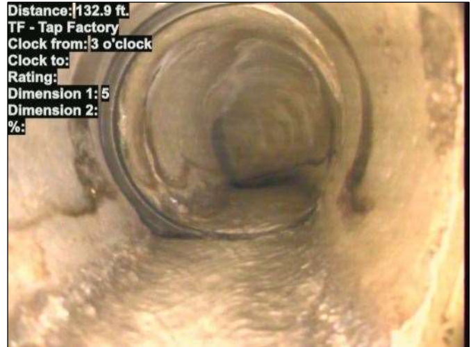
Photo: 15_047-15_048-20230725-093708.JPG At: 132.9 ft. 3/. TF - Tap Factory Joint: No
