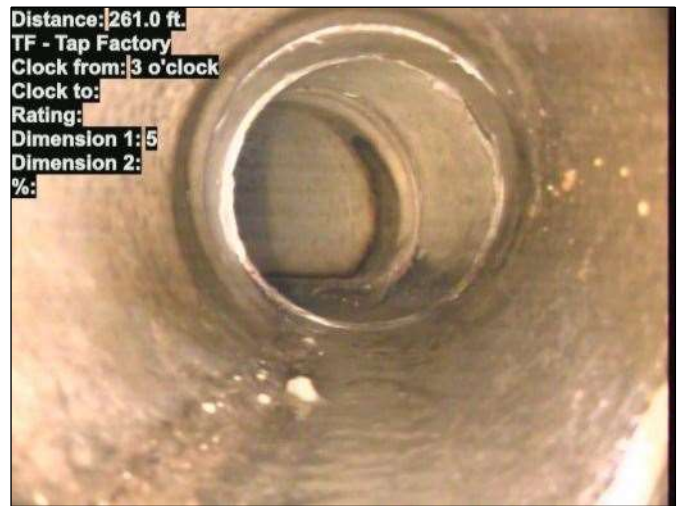
Photo: 15_027-15_026-20230725-183629.JPG At: 261 ft. 3/. TF - Tap Factory Joint: No
