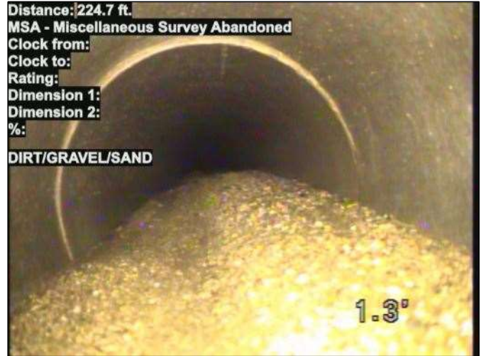
Photo: STUB-15_012-20230807-122406.JPG At: 224.7 ft. MSA - Miscellaneous Survey Abandoned Joint: No DIRT/GRAVEL/SAND
