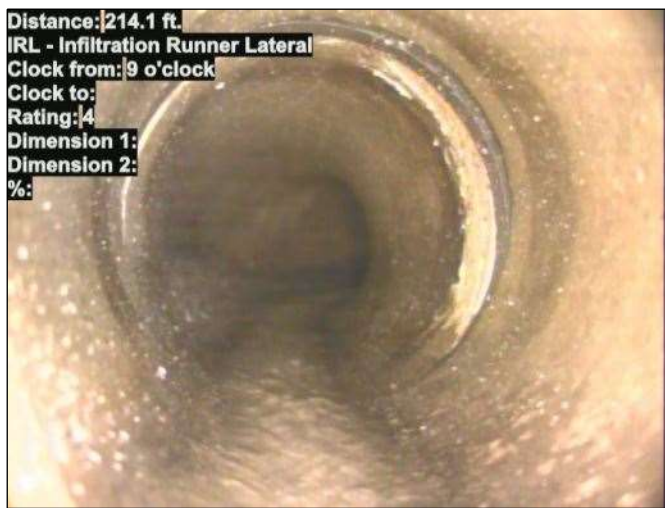
Photo: 15_042-15_043-20230801-131230.JPG At: 214.1 ft. 9/. IRL - Infiltration Runner Lateral Joint: No
