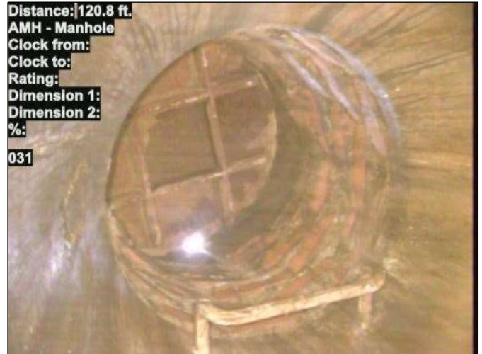
Photo: 15_030-15_031-20230724-165551.JPG At: 120.8 ft. AMH - Manhole Joint: No 031
