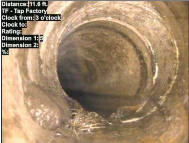
Photo: 15_031-15_032-20230724-165831.JPG At: 11.6 ft. 3/. TF - Tap Factory Joint: No
