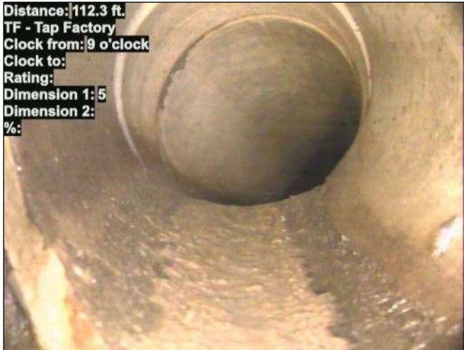
Photo: 15_047-15_048-20230725-093618.JPG At: 112.3 ft. 9/. TF - Tap Factory Joint: No
