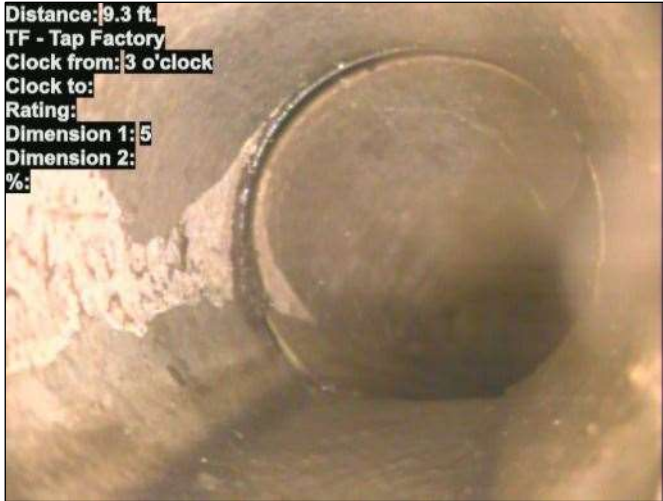
Photo: 15_079-15_078-20230801-081157.JPG At: 9.3 ft. 3/. TF - Tap Factory Joint: No
