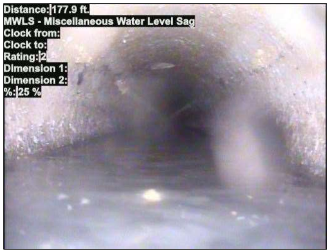
Photo: 15_059-15_060-20230804-085751.JPG At: 177.9 ft. MWLS - Miscellaneous Water Level Sag Joint: No 25 %
