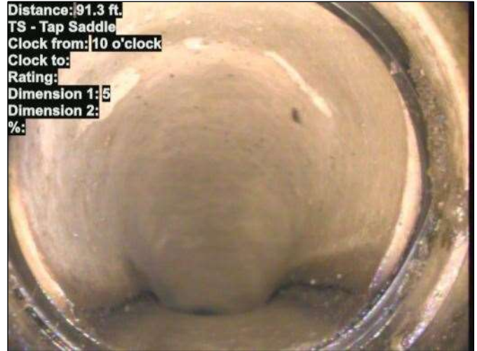
Photo: 15_038-15_039-20230724-123536.JPG At: 91.3 ft. 10/. TS - Tap Saddle Joint: No
