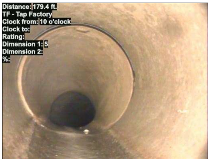
Photo: 15_046-15_047-20230725-092829.JPG At: 179.4 ft. 10/. TF - Tap Factory Joint: No
