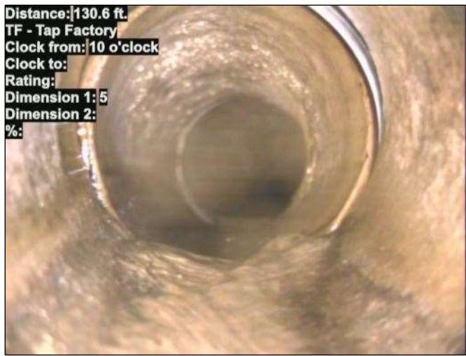
Photo: 15_022-15_023-20230724-154854.JPG At: 130.6 ft. 10/. TF - Tap Factory Joint: No
