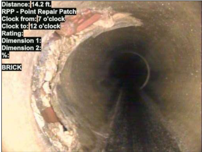
Photo: 15_002-15_003-20230725-112219.JPG At: 14.2 ft. 7/12 RPP - Point Repair Patch Joint: No BRICK
