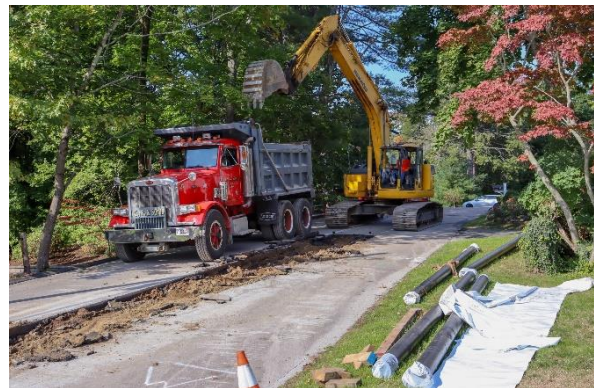
Hillcrest Place is being dug for a new water main.
