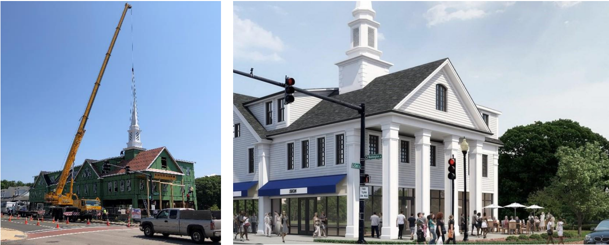
Mixed-use Building at 282-298 Washington Street
