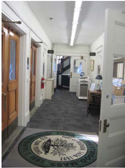
View of the front lobby with painted walls and ceilings and recently (2015) installed carpet tile flooring.
