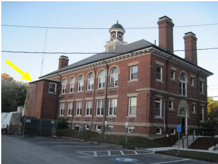
View of the rear (east) and north end elevations. Note egress stairwell addition (arrow) constructed at an unknown later date in order to comply with local minimum egress requirements.
