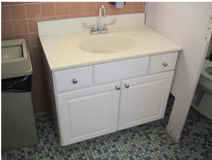
View of older fixtures and finishes within the first floor women's restroom.
