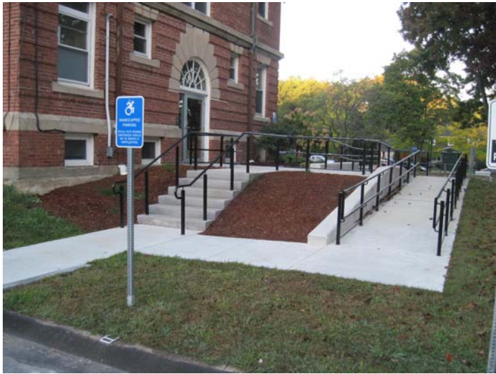
View of the recently installed concrete accessible entrance ramp, stairs, and painted steel tube railing.
