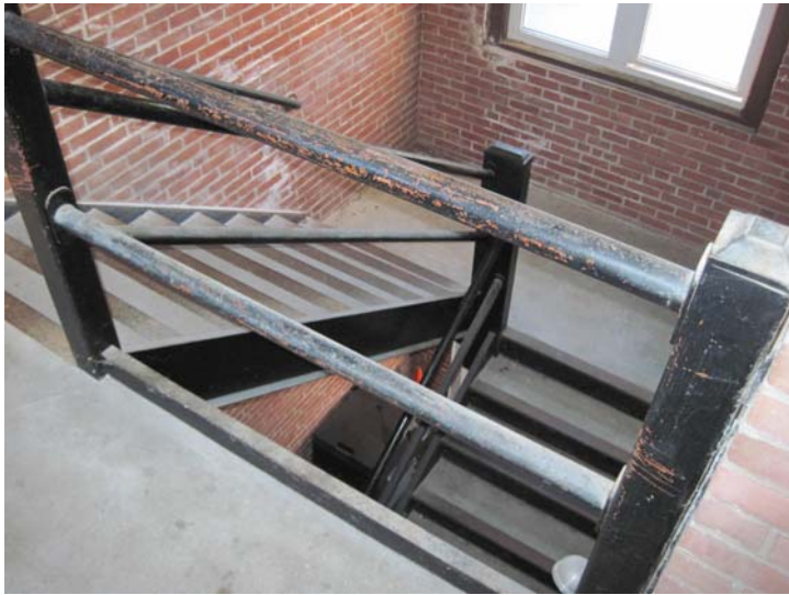
View of the brick-enclosed, rear elevation, concrete and steel, secondary egress stairwell.
