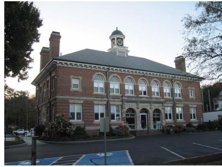
View of the building front (west) elevation with mix of face-brick; cast-stone lintels, sills, and trim elements; recently repainted wood dentil block soffits, older three-tab asphalt shingle roof, and copper-domed cupola with four-sided clock.
