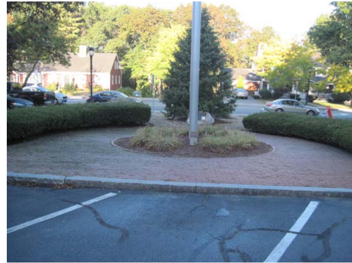
View of the laid brick walkway and landscaping surrounding the front elevation flag pole.
