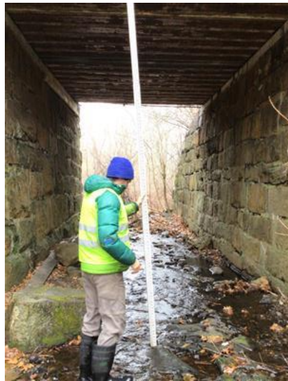
Culvert inspection in Walpole
