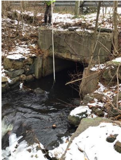
Culvert inspection in Sharon
