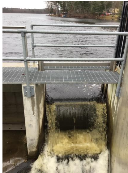
Dam inspection in Canton
