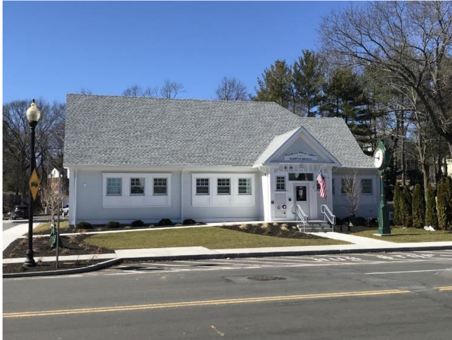
Relocated Wentworth Hall, Washington St. Islington Home of the new Islington Library
