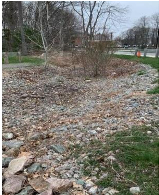
Image of the Deerfield Avenue Infiltration Basin from an August, 2022 MS4 inspections. This is an example of a Best Management Practice to reduce the pollutants in stormwater runoff, and to reduce localized flooding.
