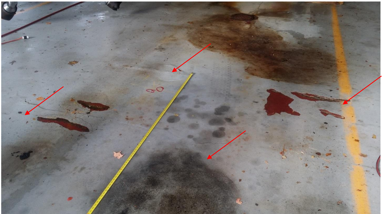
Photo 2 – Minor cracking on the top of the elevated slab.
