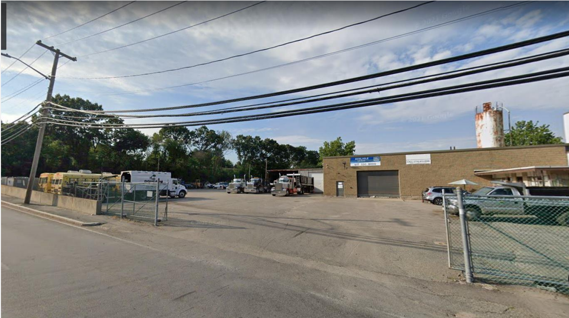
Foster Block Property - 22 Everett Street capacity for 102 housing units
