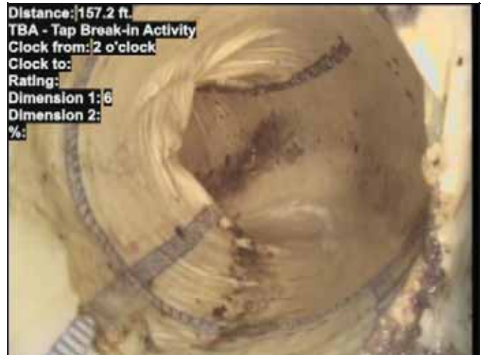
Photo: 16_067-16_068-04302020-TBA-157.2 ft.-112414.JPG At: 157.171 ft. TBA - Tap Break-in Activity Joint: No 2/.
