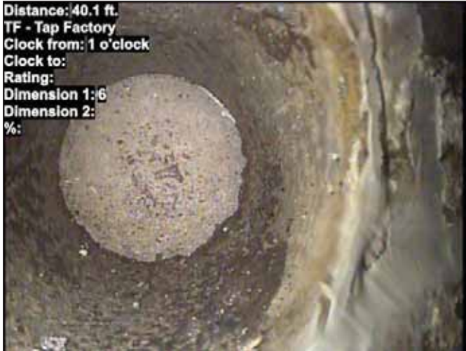
Photo: 14_013-14_017-20181116-090913.JPG At: 40.1 ft. 1/. TF - Tap Factory Joint: No
