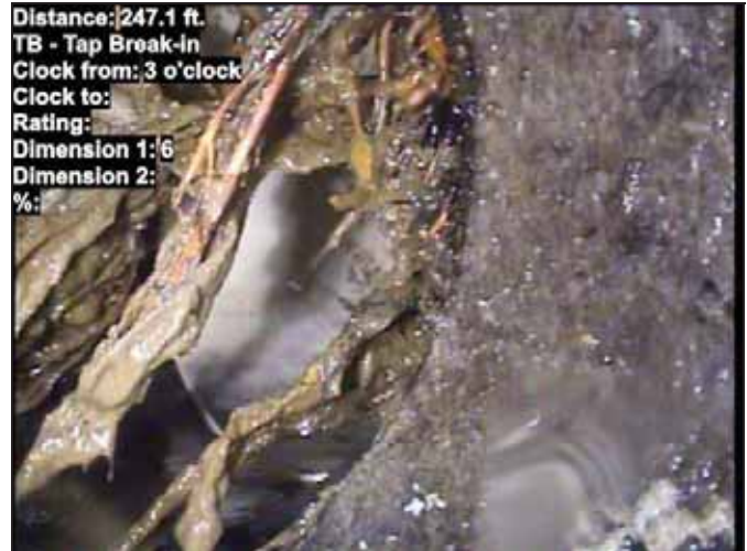
Photo: 14_013-14_017-20181116-093734.JPG At: 247.1 ft. 3/. TB - Tap Break-in Joint: No
