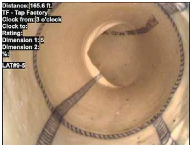
Photo: 10_078-10_079-20191226-140625-141524.JPG At: 165.6 ft. 3/. TF - Tap Factory Joint: No LAT#9-5
