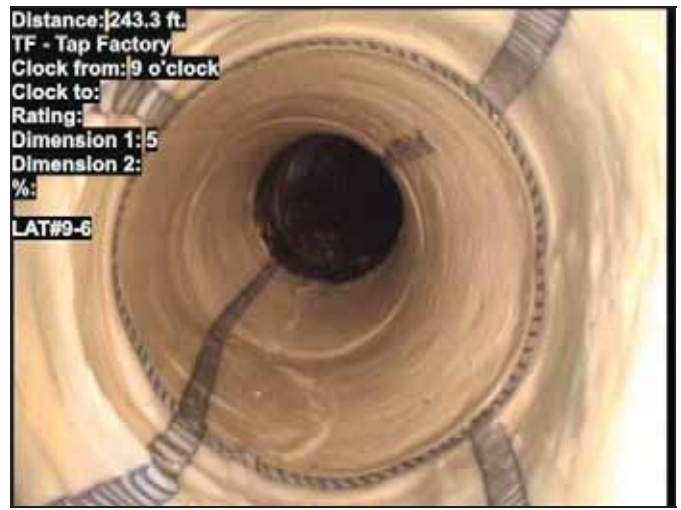
Photo: 10_078-10_079-20191226-140625-141827.JPG At: 243.3 ft. 9/. TF - Tap Factory Joint: No LAT#9-6
