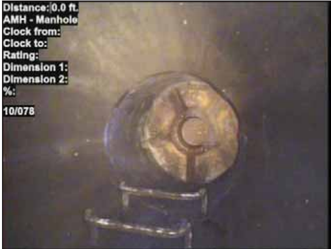
Photo: 10_078-10_079-04292020-AMH-0.0 ft.-120709.JPG At: 0 ft. AMH - Manhole Joint: No 10/078
