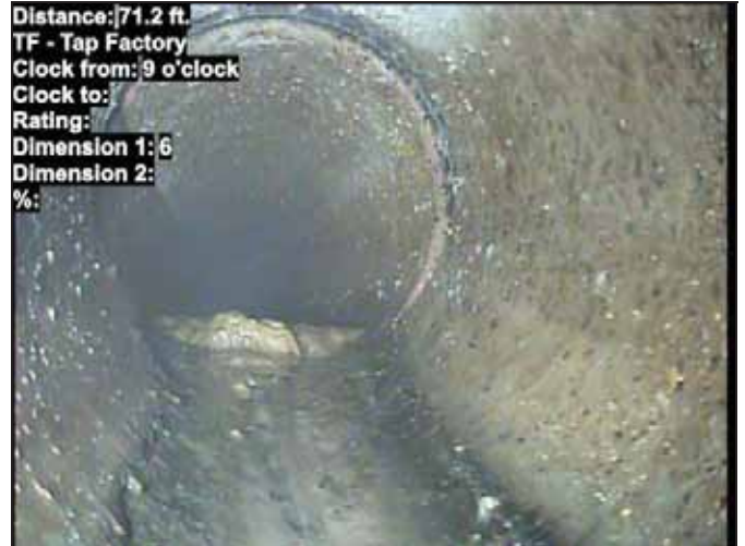
Photo: 14_070-14_071-20181116-115613.JPG At: 71.2 ft. 9/. TF - Tap Factory Joint: No
