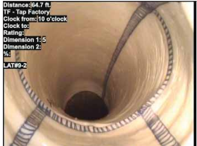
Photo: 10_078-10_079-20191226-140625-141103.JPG At: 64.7 ft. 10/. TF - Tap Factory Joint: No LAT#9-2
