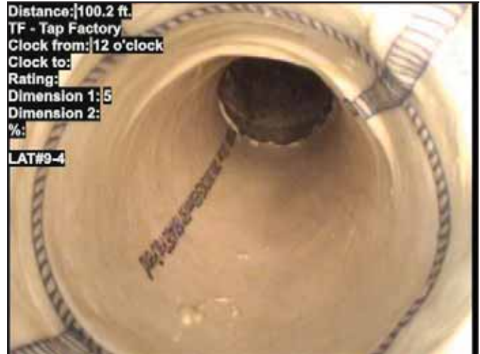
Photo: 10_078-10_079-20191226-140625-141303.JPG At: 100.2 ft. 12/. TF - Tap Factory Joint: No LAT#9-4
