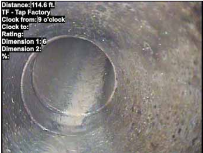
Photo: 14_070-14_071-20181116-115742.JPG At: 114.6 ft. 9/. TF - Tap Factory Joint: No
