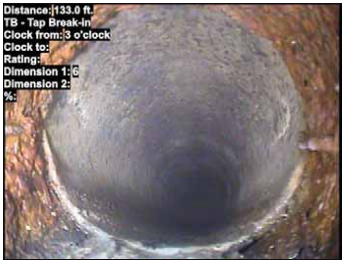
Photo: 14_070-14_071-20181116-115834.JPG At: 133 ft. 3/. TB - Tap Break-in Joint: No
