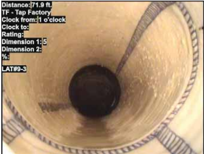
Photo: 10_078-10_079-20191226-140625-141144.JPG At: 71.9 ft. 1/. TF - Tap Factory Joint: No LAT#9-3
