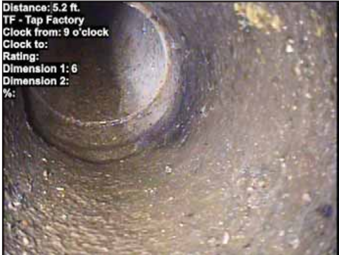
Photo: 14_070-14_071-20181116-115427.JPG At: 5.2 ft. 9/. TF - Tap Factory Joint: No
