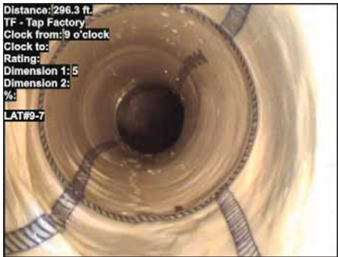
Photo: 10_078-10_079-20191226-140625-142044.JPG At: 296.3 ft. 9/. TF - Tap Factory Joint: No LAT#9-7
