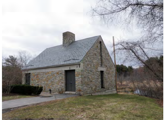
Sewer Pump Station located at Conant Road
