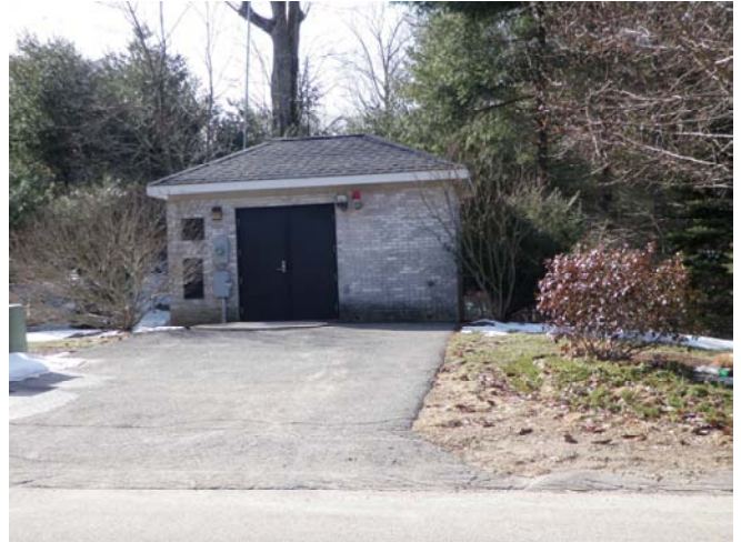
Sewer Pump Station located at Stonemeadow Drive
