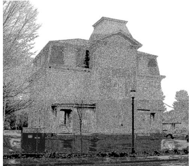
The Colburn School with Mansard roof and Plexiglas window protection completed in 2007.
