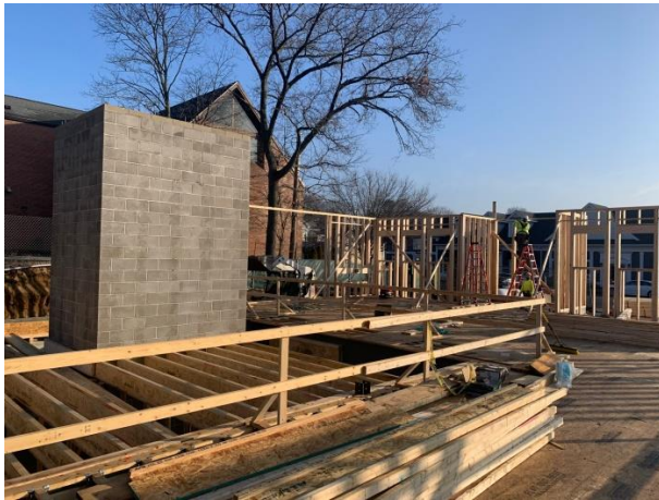
Photos showing completed elevator shaft and wood framing at the New Wentworth Hall
