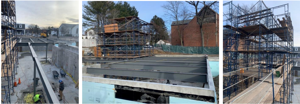
Photos showing steel framing and staging for elevator shaft at the New Wentworth Hall
