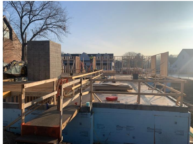
Photos showing completed elevator shaft and wood framing at the New Wentworth Hall
