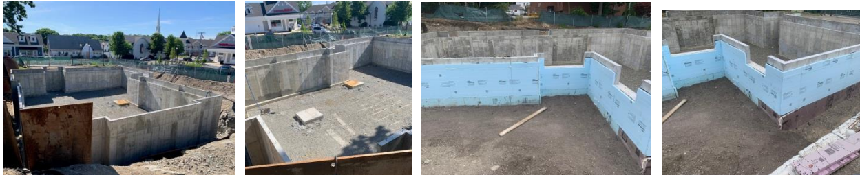
Photos showing construction of foundation for New Wentworth Hall
