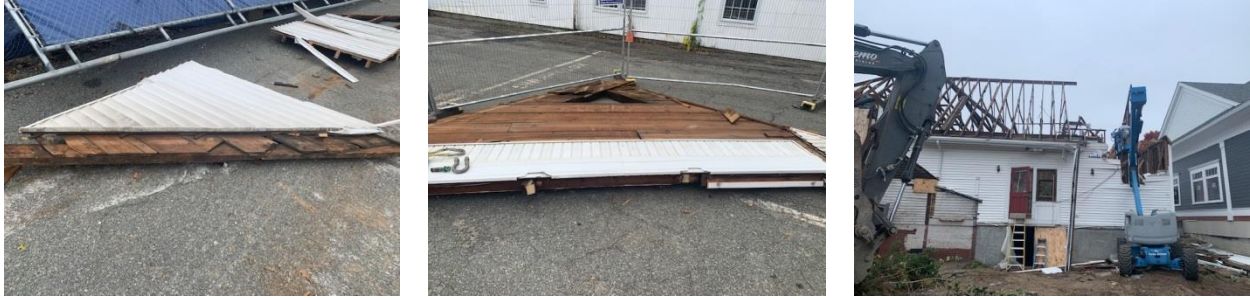
Photos showing removal of wall panels from Old Wentworth Hall for incorporation in New Wentworth Hall
