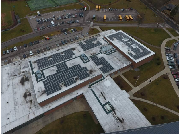
Solar at Westwood High School
