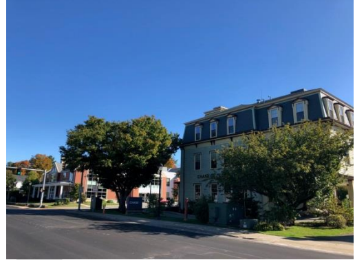
Historic Colburn School on High St.
