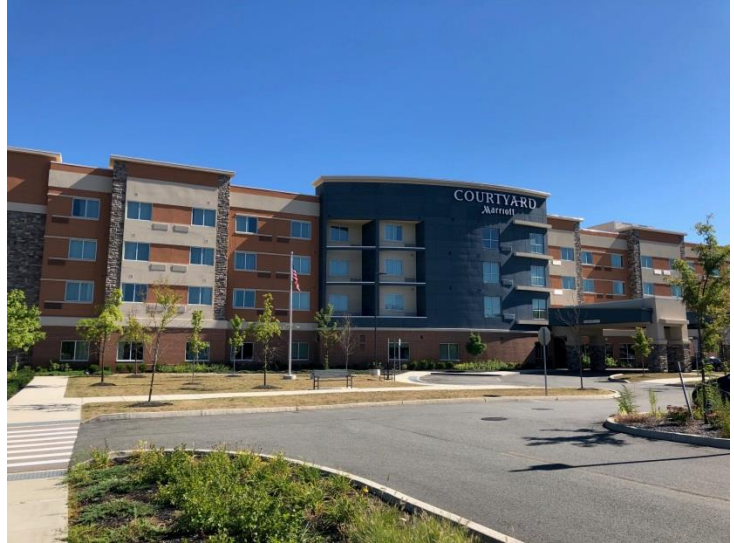
Courtyard Marriott, University Station
