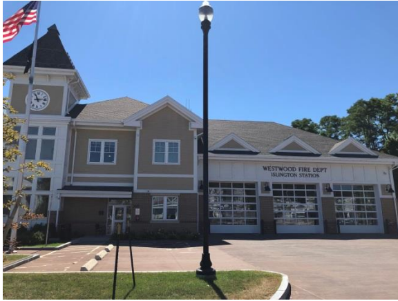
Islington Fire Station
