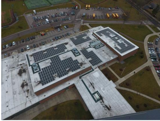
Solar at Westwood High School
