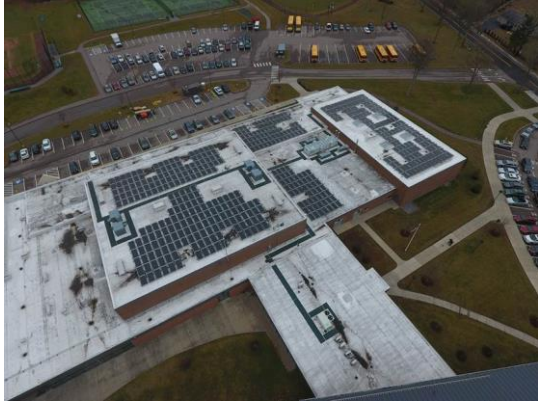
Solar at Westwood High School
