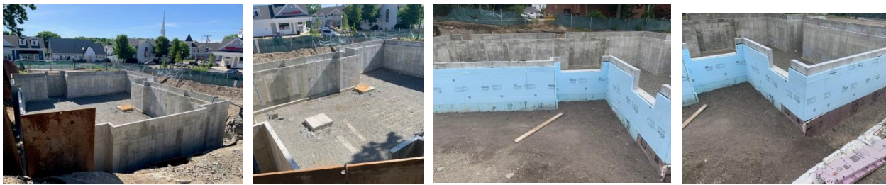
Photos showing construction of foundation for New Wentworth Hall
