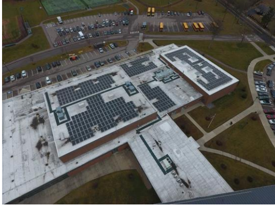
Solar at Westwood High School
