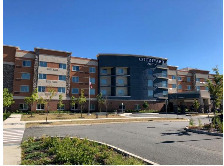
Courtyard Marriott, University Station
