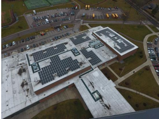
Solar at Westwood High School
