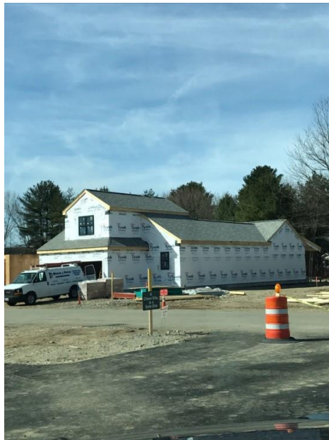
Condo construction at the former Westwood Lodge
