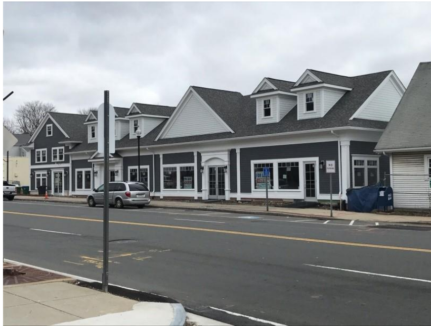
Commercial renovation at the former CVS building on Washington Street
