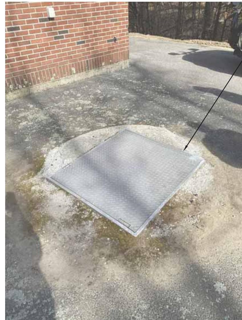
P1: WET WELL TOP SLAB
