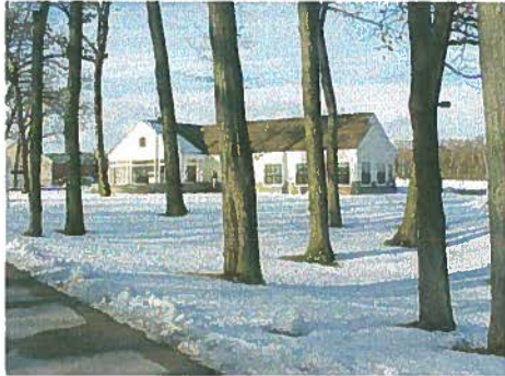
Westwood's Senior Center Constructed in 1999
