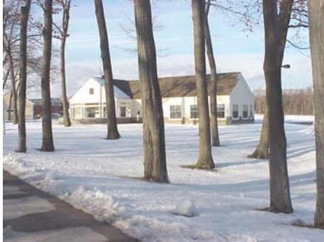
Westwood's Senior Center Constructed in 1999
