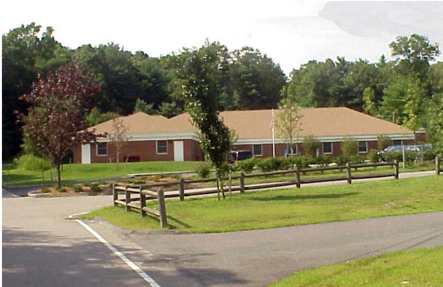
New Municipal Office Building Completed July, 2004
