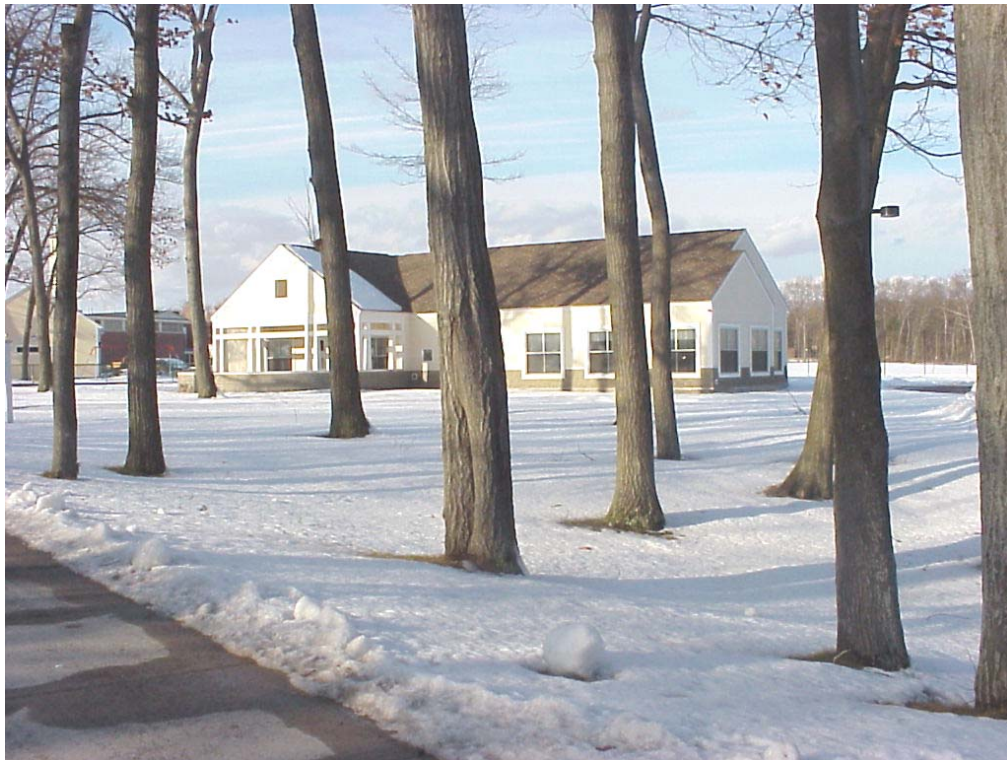
Westwood's Senior Center Constructed in 1999
