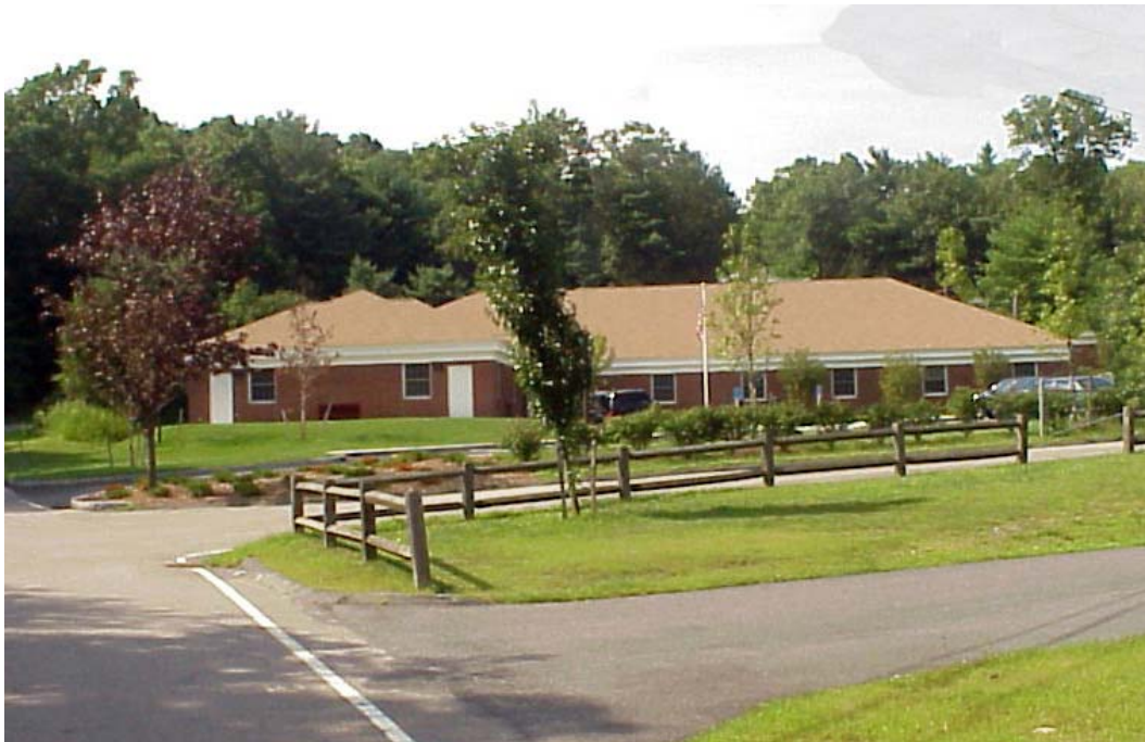
Carby Street Municipal Office Building
