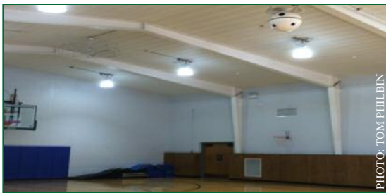
Lighting Upgrades at Downey Elementary School Gymnasium
