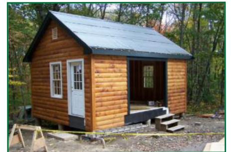
Boathouse, under construction, at Noanet Landing.
